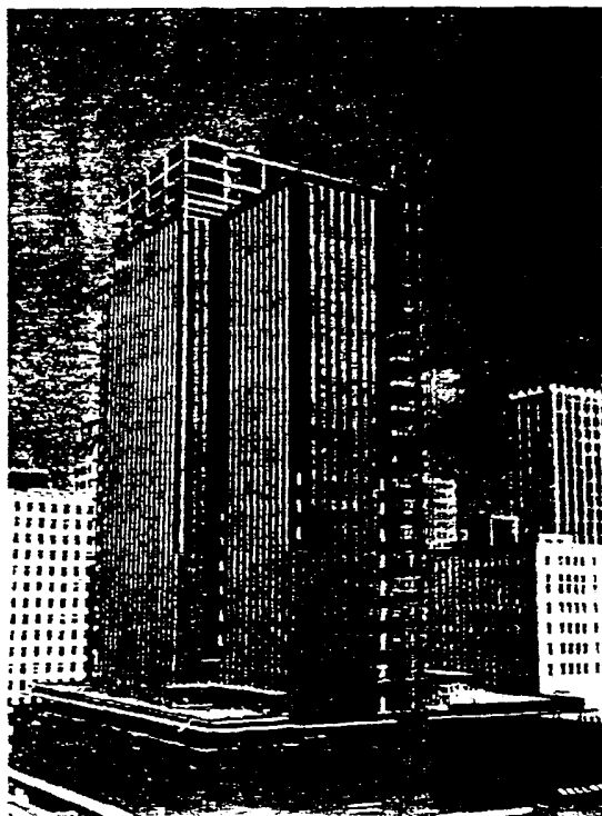
Maroon strips of porcelain enamel run twenty stories high and set off the aluminum skin of the Second National Bank Building in Houston, Tex.
