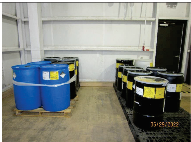
Photograph #14 – Permitted Storage Building (b) (3) (A) - Seven 55-gallon containers storing hazardous waste (left side) in the General Waste Cell. Two 55-gallon containers and six 35-gallon containers of hazardous waste (right side).
