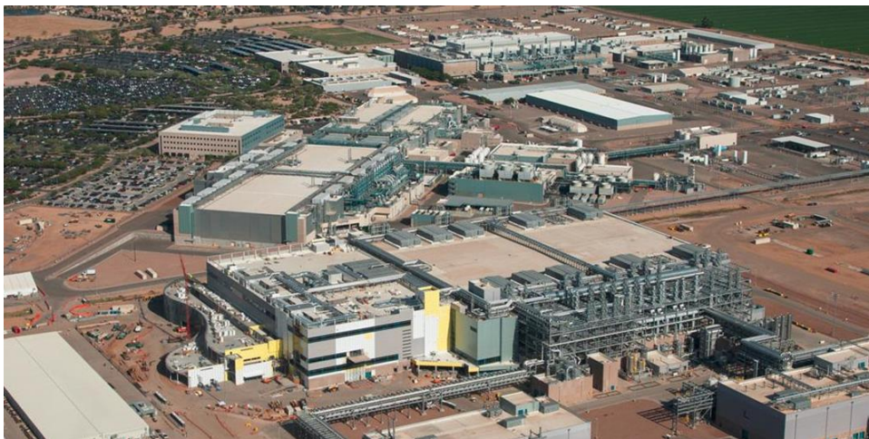
Figure 18: A semiconductor manufacturing facility (Intel 2017).
