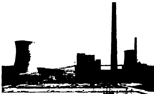
Big Sandy Station No. 2 of Kentucky Power Company, housing a 737,000-kw double reheat turbine.
