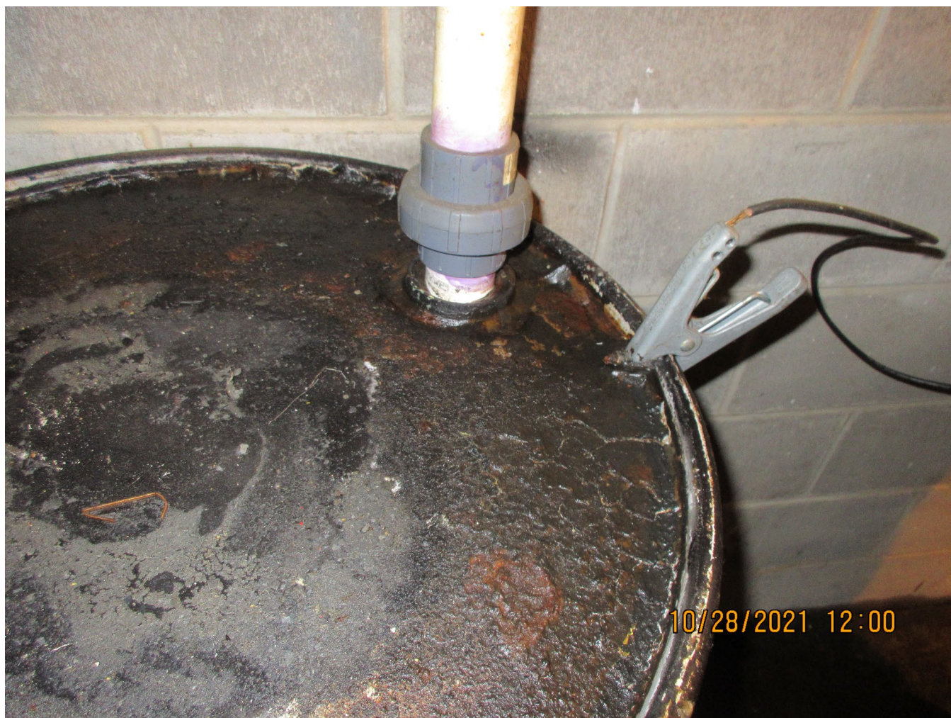
Photo 24 – Unsealed container hazardous waste in SAA # 14 (Solvent Room)
