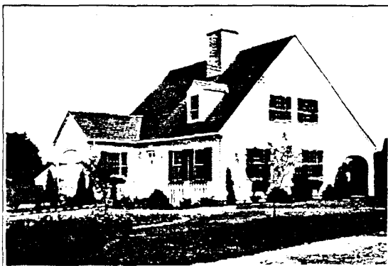
COURTESY GENERAL ELECTRIC CO.
