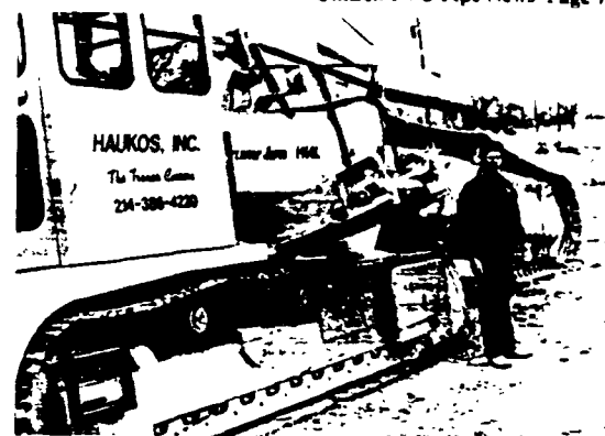
The trenching machine speeds up construction.
