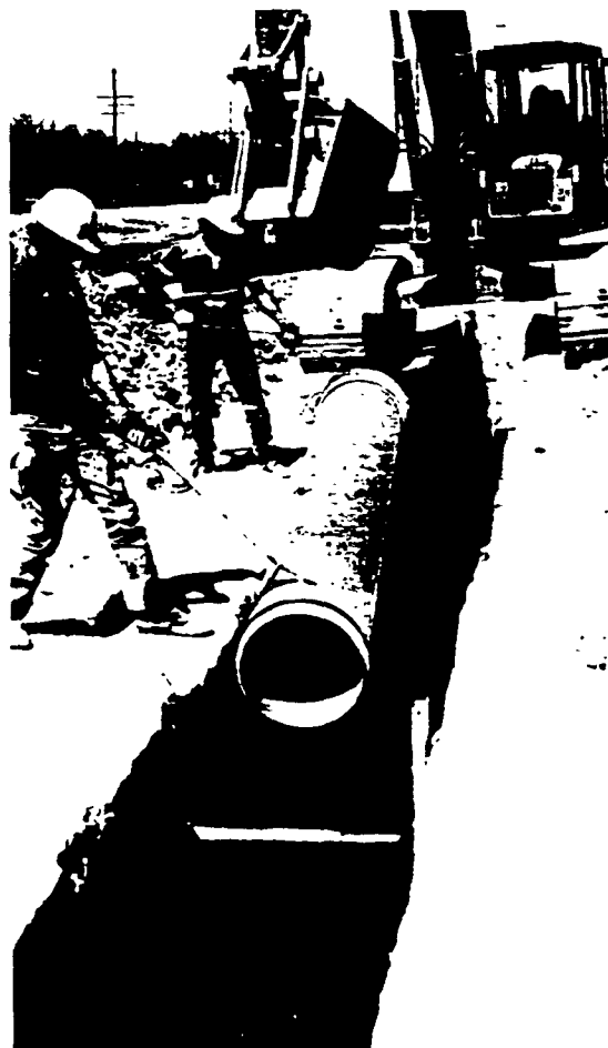
The light-weight PVC is manhandled.
