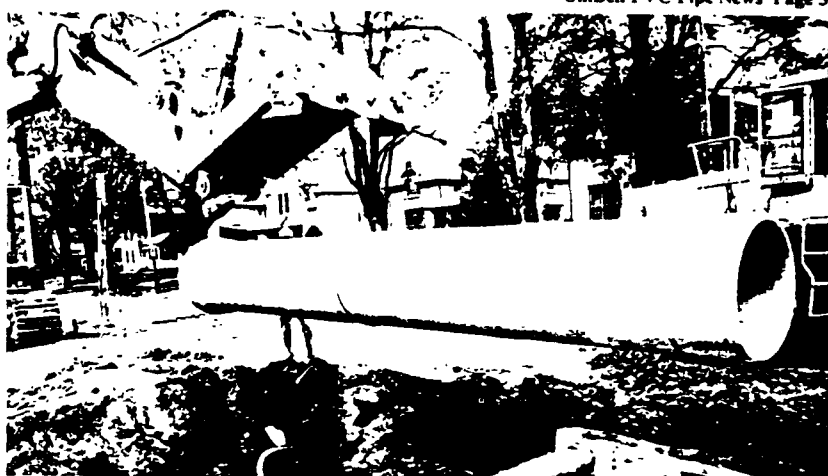
The 20-foot length of 30-inch PVC is handled with light-weight equipment.
