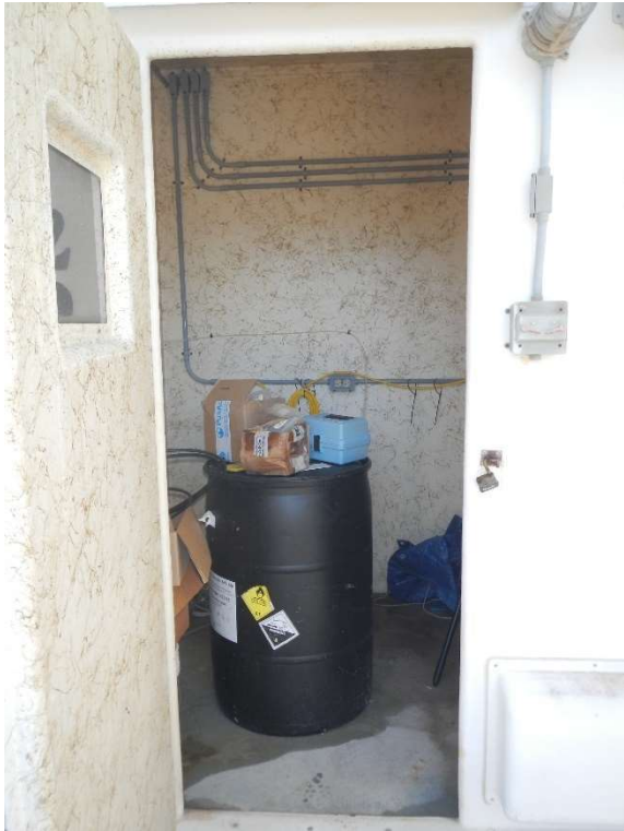
Photograph 1: Water Treatment Plant Storage Area
