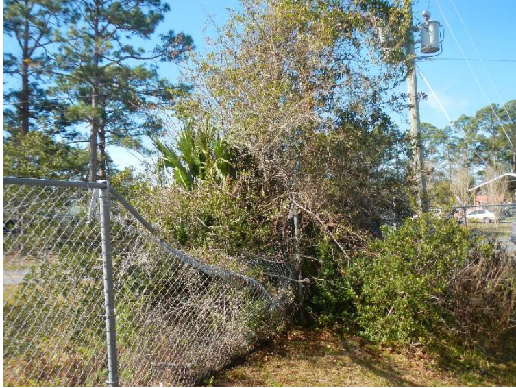
Photograph 4: Vegetation on Water Treatment Plant fence
