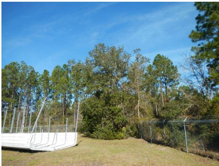
Photograph 5: Vegetation on Water Treatment Plant fence
