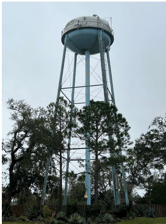
Photograph 18: Branches touching support structure Provided by FDEP staff – taken on February 3, 2022
