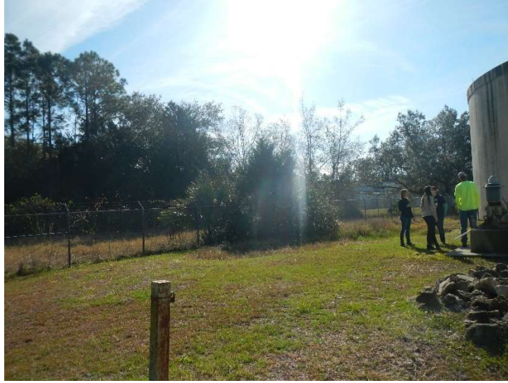
Photograph 6: Vegetation on Water Treatment Plant fence
