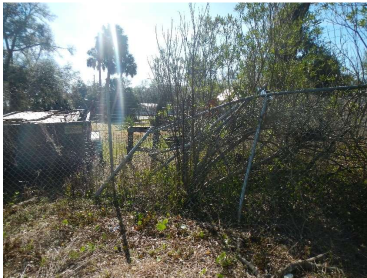
Photograph 7: Vegetation on Elevated Storage Tank fence
