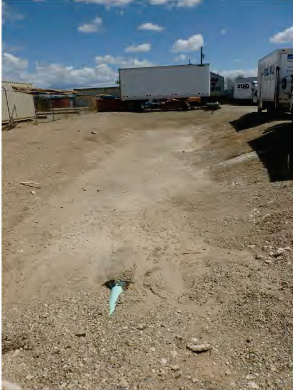
Photo 1 / P1000866 – Detention Pond, NE detention pond
