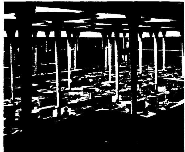
Striking interior of the Johnson office building, showing the unique column design and glass tubing ceiling behind which the lights are concealed
