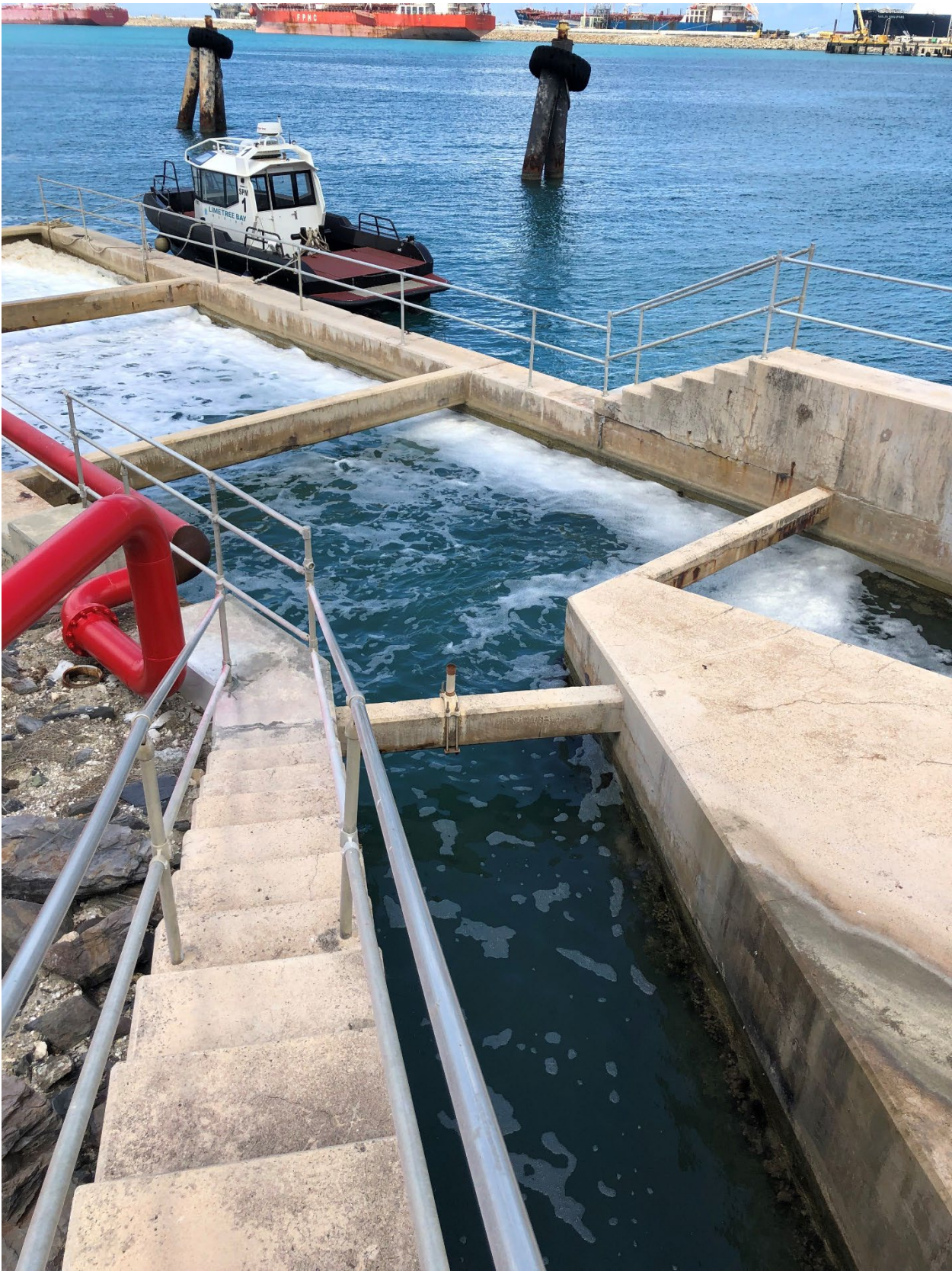
Photo #5: Seawater Intake.
