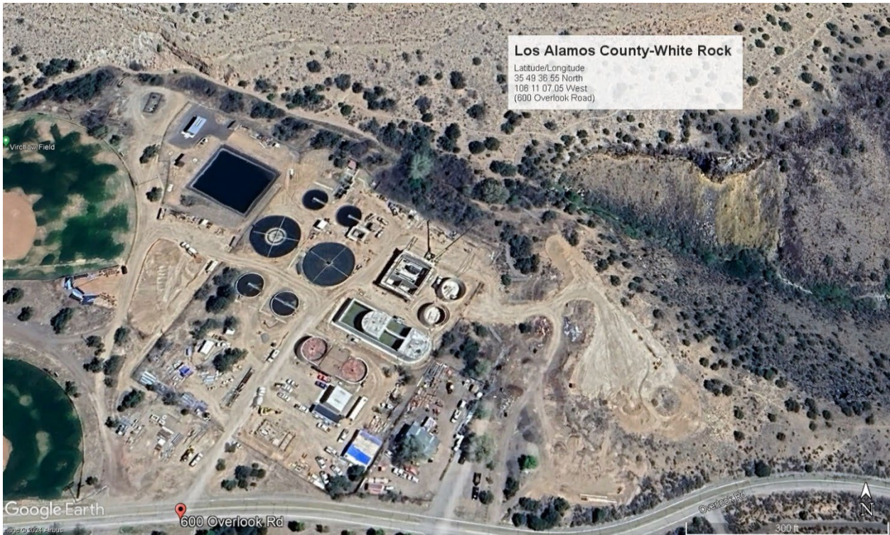
Aerial Image #1: Overall view of the Los Alamos-White Rock Wastewater Treatment Facility. Note: this Aerial Image is dated May 7, 2023, and illustrates the existing WWTF. Aerial from Google Earth maps.
