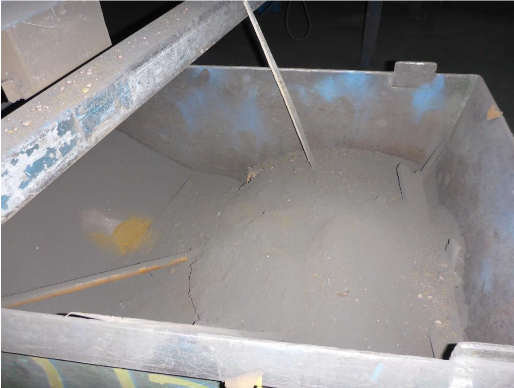
Photo 14: Metal hopper for accumulating separated material that has been processed in the Reclaim Room. The hopper is labeled D008 hazardous waste 02/08/2021 and appears to contain used foundry sand.
