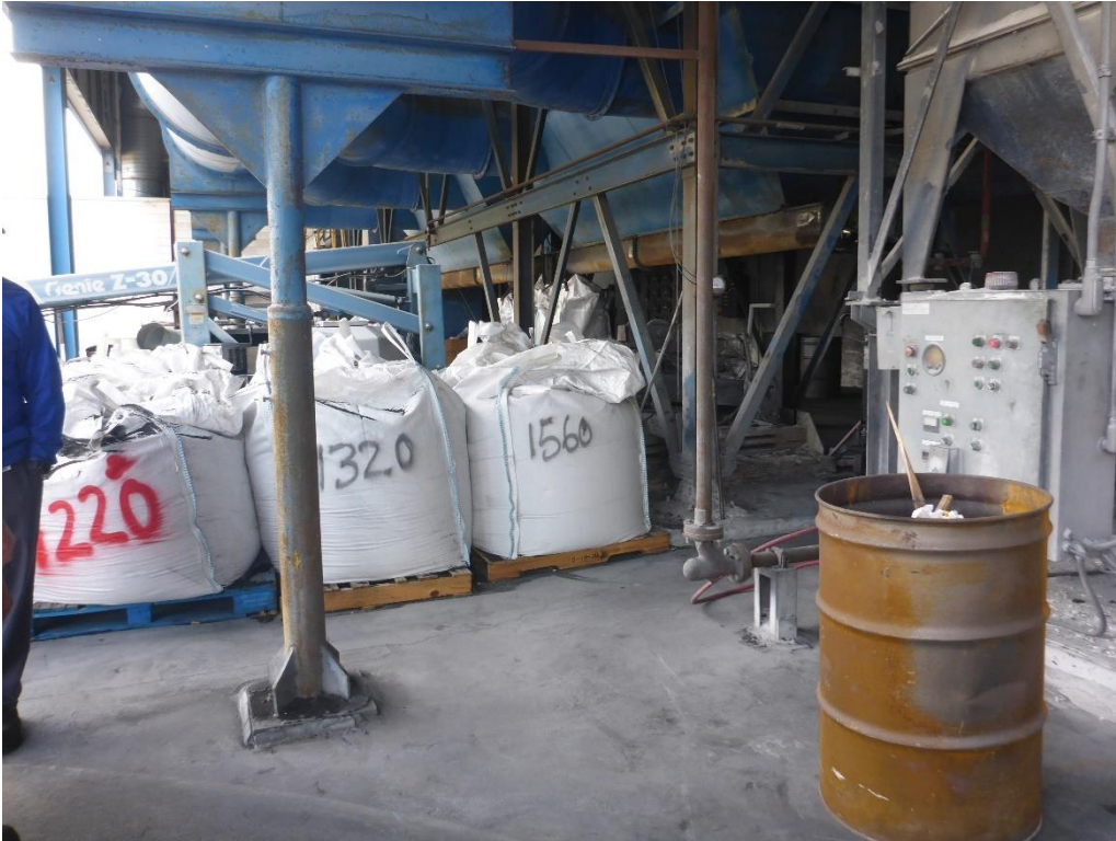
Photo 31: Supersacks observed in the Baghouse area. Bags were not labeled, but facility personnel stated they contain zinc material that will be sold for use off-site. Spray painted numbers indicate the weight of the bag.
