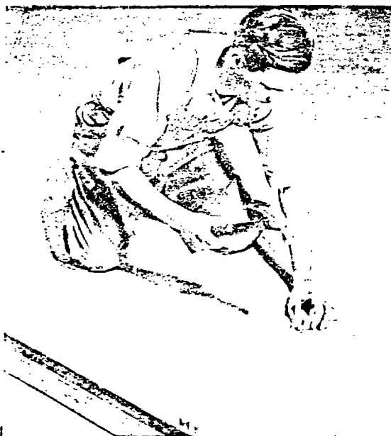
FIRST, nail down metal floor clips approximately 24 inches on center. The metal base side plates snap over shoulders of clips. Then grout gypsum plaster into base section.
