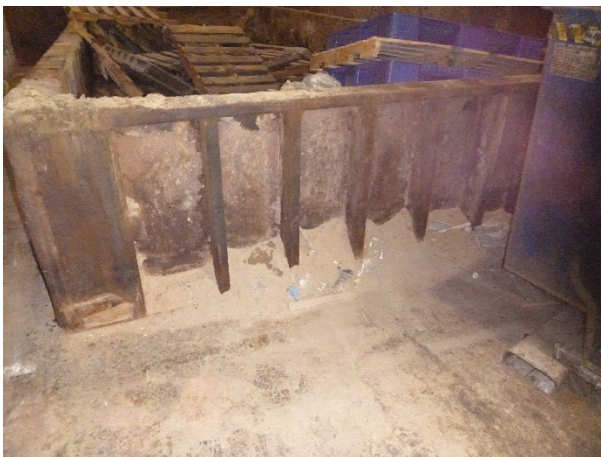
Photograph 36: Building 3 treatment pan.
