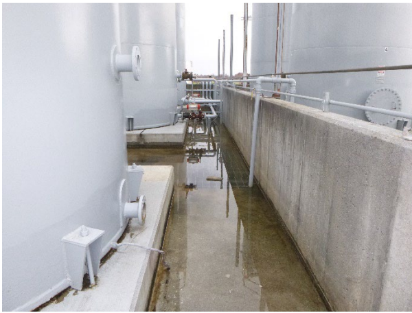
Photograph 46: Tank Farm Secondary Containment.
