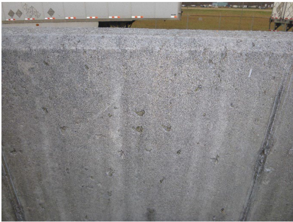
Photograph 47: Tank Farm Secondary Containment.
