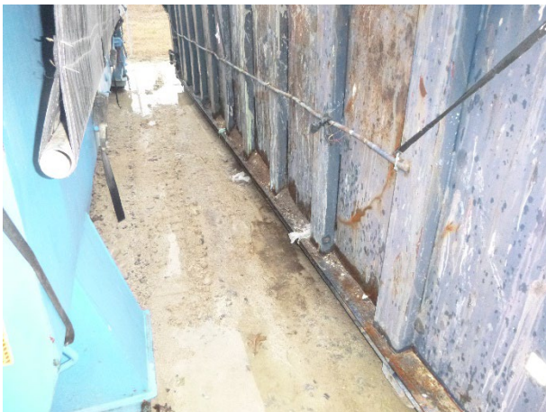
Photograph 48: Building 3 waste staged for processing in Building 3.
