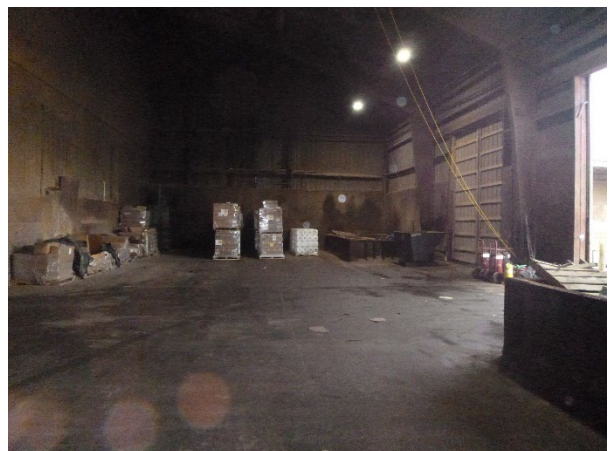
Photograph 33: Building 3 treatment pan.
