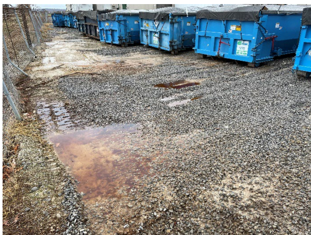
Photograph 52: CAA behind Building 3.
