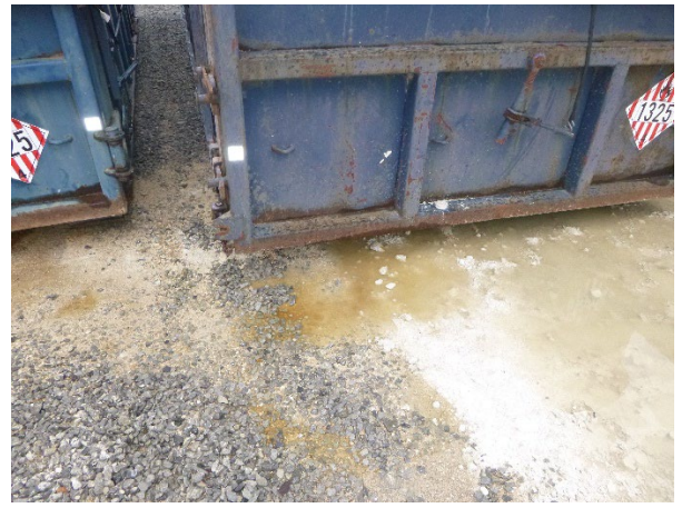
Photograph 51: CAA behind Building 3.
