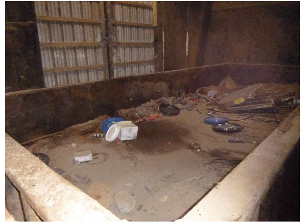
Photograph 38: Building 3 treatment pan.
