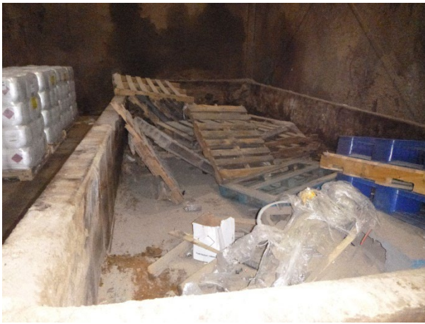
Photograph 34: Building 3 treatment pan.
