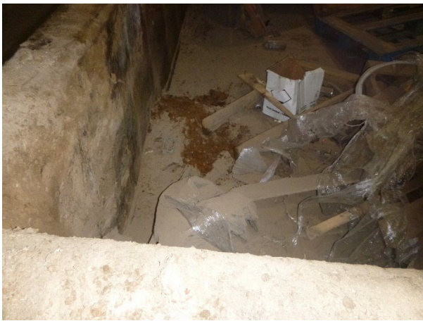
Photograph 35: Building 3 treatment pan.
