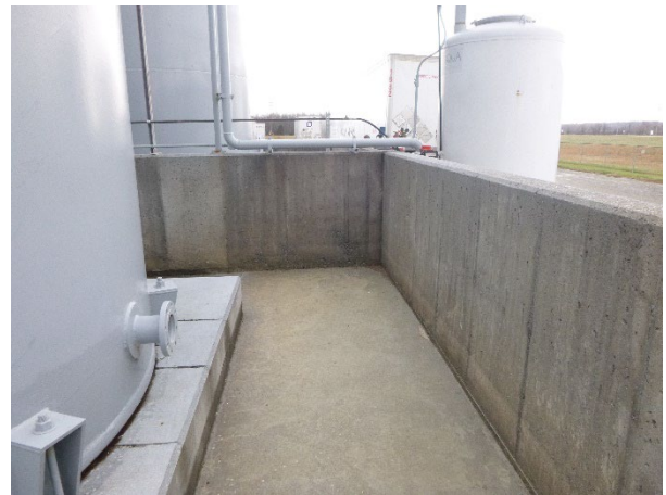
Photograph 45: Tank Farm Secondary Containment.
