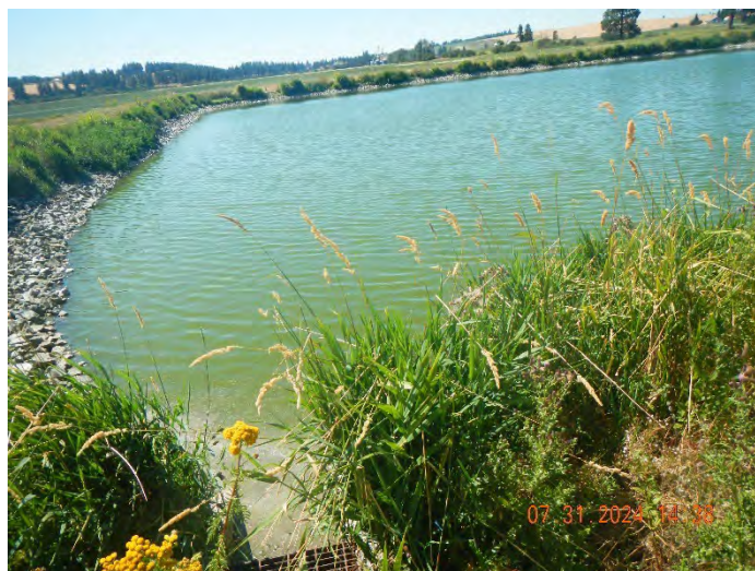
Photo #:07 (DSCN3861) Description: Facing west, photo of Lagoon 2 discharge to the chlorine mixing box.
