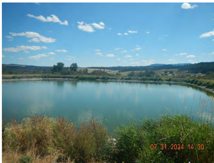
Photo #:04 (DSCN3858) Description: Facing south, photo of Lagoon 2.
