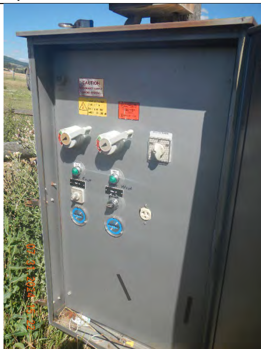
Photo #:18 (DSCN3872) Description: Photo of pump meter display for Lift Station 1.
