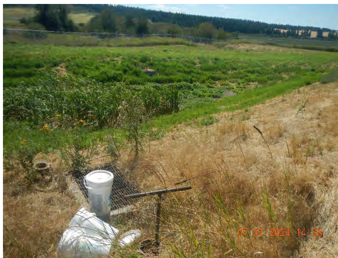
Photo #:08 (DSCN3862) Description: Facing southwest, photo of the chlorine mixing box.
