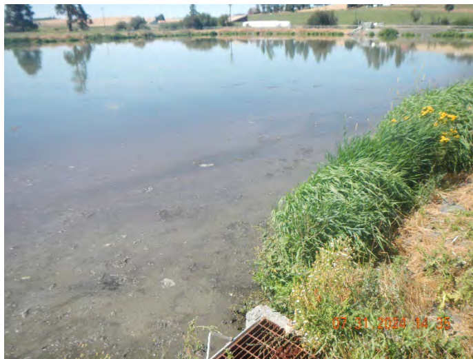
Photo #:06 (DSCN3860) Description: Facing northwest, photo of Lagoon 2 bypass structure.
