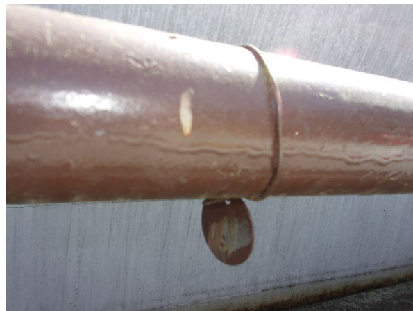
Figure 18: 10:38 AM Tank Farm
