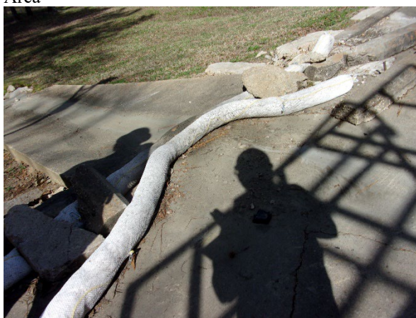
Figure 28: 10:17 AM Non-Hazardous Waste Frac Tank Area
