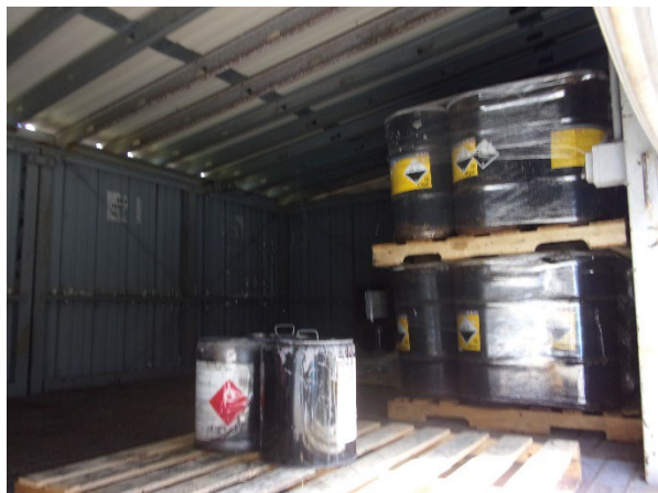
Figure 31: 10:20 AM Flammable Storage Shelter
