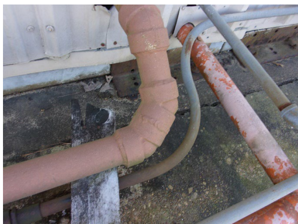
Figure 21: 10:37 AM Tank Farm
