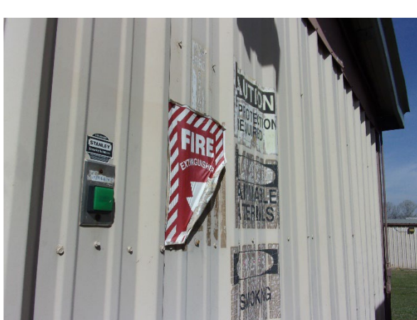
Figure 30: 10:20 AM Flammable Storage Shelter
