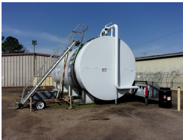
Figure 32: 10:25 AM Used Oil Tank Area
