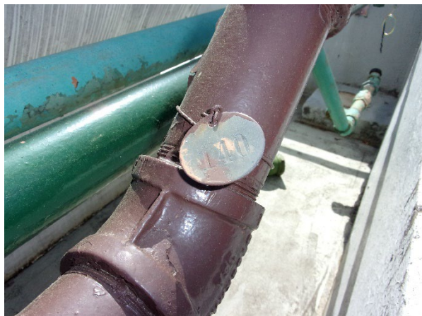
Figure 19: 10:38 AM Tank Farm
