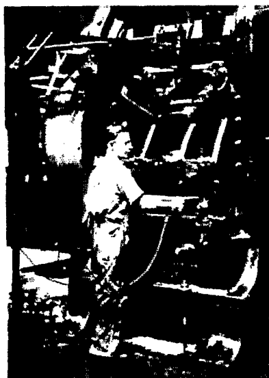
When the ram of the press descends the operator's hands are pulled back from the danger zone.
