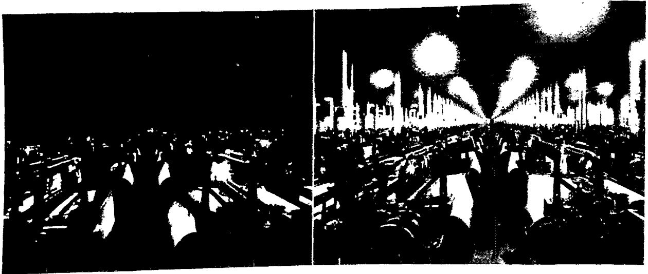
Figures 3 and 4. At the left is a textile mill illuminated only by direct lighting. At the right is the same room provided with adequate light well diffused and distributed.
