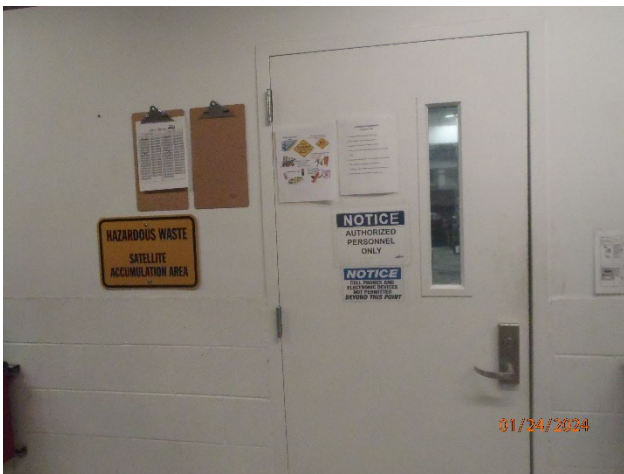
Picture 7 – Paint Kitchen 2 SAA entrance
