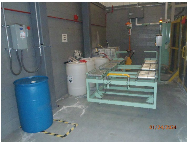
Picture 13 – Electro Clean Storage
