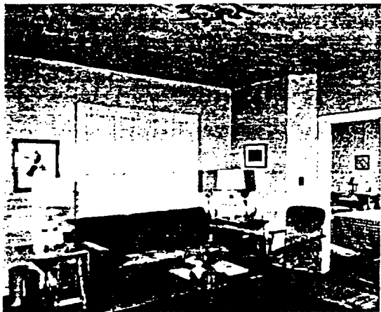
Before. Just a thoroughfare between other rooms was this old living room, connecting directly to a bedroom and stairway. Note the cracked ceiling, battered woodwork and scuffed floors.
