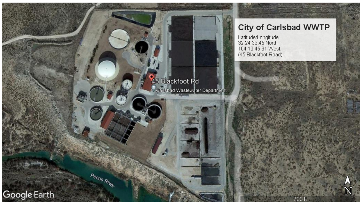
Aerial Image #1- Overall view of the City of Carlsbad Wastewater Treatment Plant. Aerial from Google Earth.
