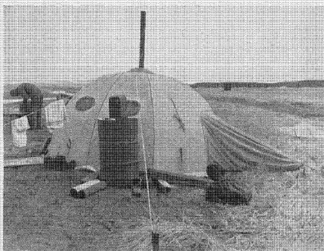
This portable shelter looks like an Eskimo's igloo, and was unharmed by 80 mph winds during tests in Aleutians.
