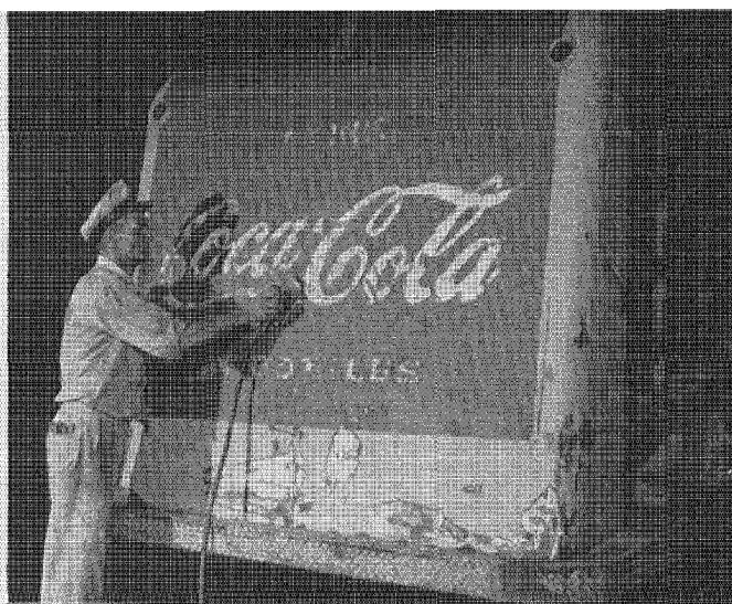
Sanding a truck to prepare it for the actual refinishing. Houston Coca-Cola repaints its trucks on regular schedule.
