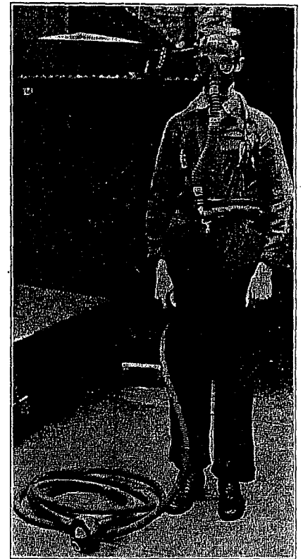
Courtesy, U. S. Bureau of Mines Fig. 6. Hose mask with Tissot face piece. A helmet can be used instead of a face piece, but the latter is now preferred by most persons. The hose is strongly fastened to a wide heavy web belt, which precludes pulling the mask away from the face of the wearer.
