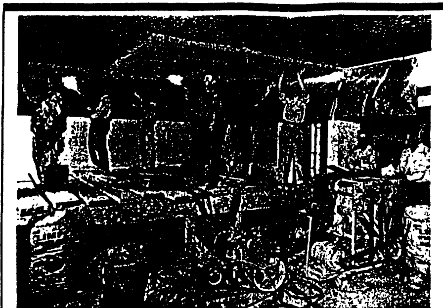
"LIMPET" sprayed asbestos application. LIMPET was a product of the Keasbey and Mattison Company. Note the two men at the far right feeding the machines. Courtesy of Mitchell Cohen.
