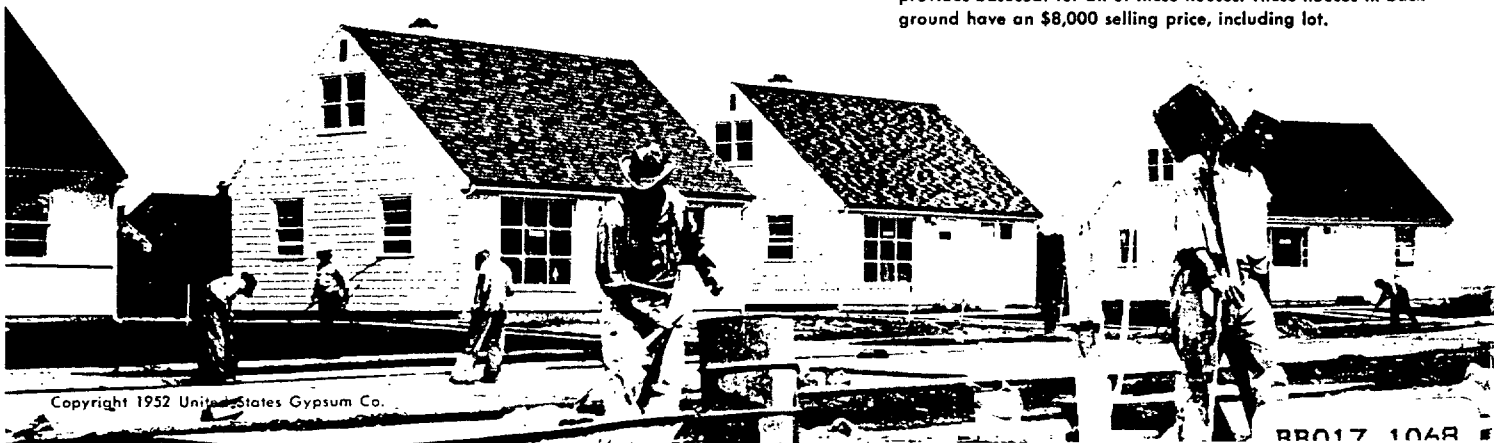
RED TOP cement plaster with perlite aggregate hand mixed provides basecoat for all of these houses. These houses in background have an $8,000 selling price, including lot.
