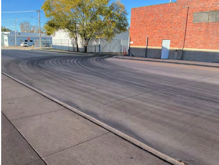
IMG_0524.JPG: This image was taken from 4th Street that shows how the trucks track spilled glycerin or Veg Oil onto the public roadway. Also shows the fire water connection on the street side that was discussed in Image 41.
