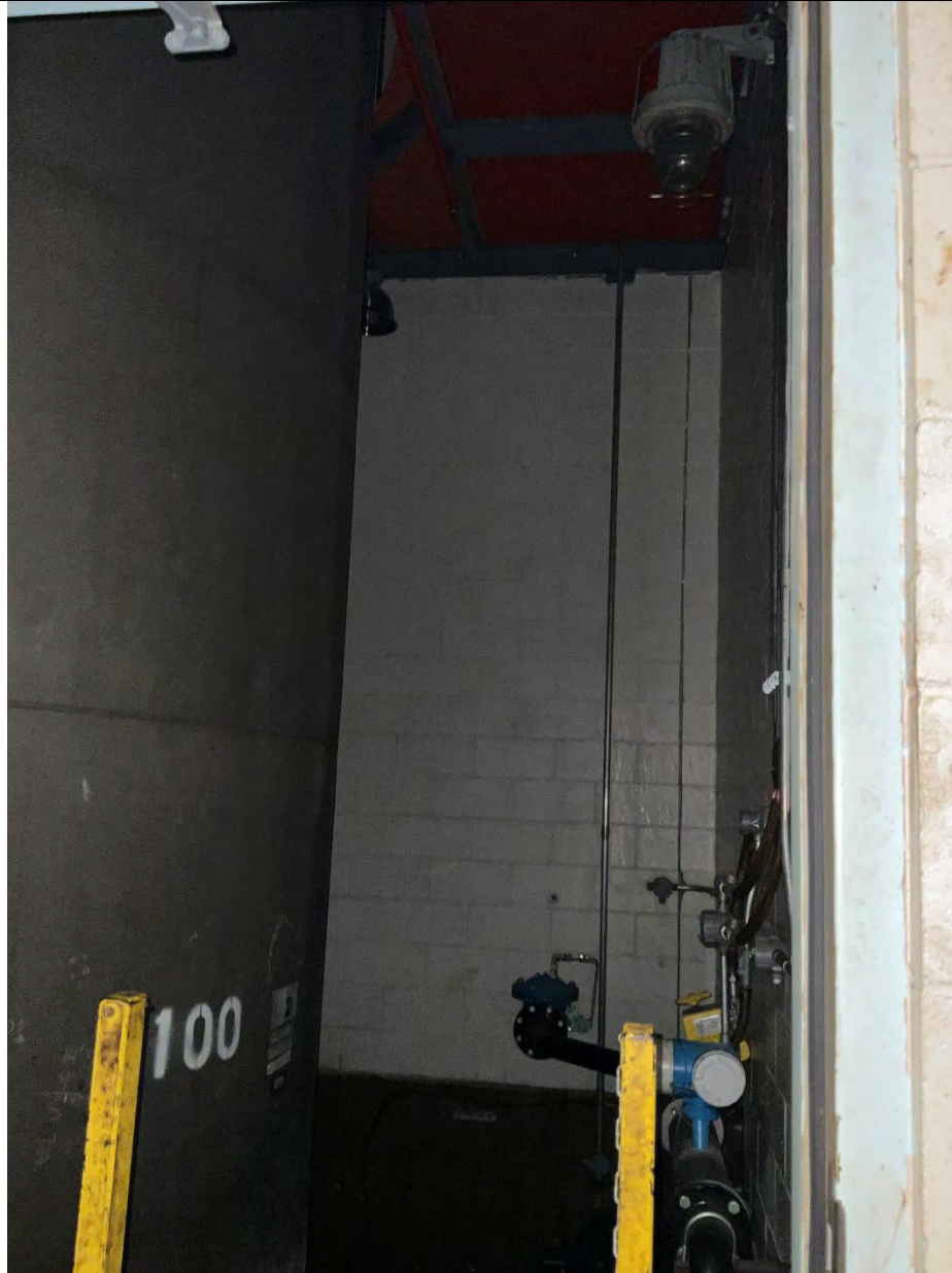
Image of room taken from outside of the confined space.
