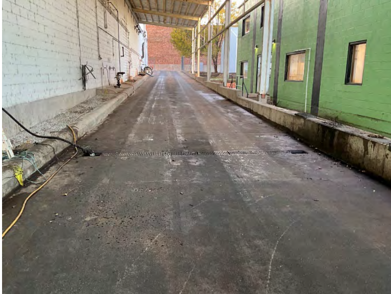
IMG_0513.JPG: Trucks that will be loaded with methanol, glycerin, or vegoil, enter from the east or from the 5th street side of the facility and pull up to the loadout areas located on the processing buildings south wall. The grate running through the driveway is where spills from truck loading are captured and then pump via sump pump into the pit as seen in Images 42 and 43.
