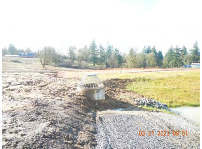
Photo #:06 (DSCN3166) Description: Facing south, photo of the overflow structures to the southern stormwater pond (Tract G).
