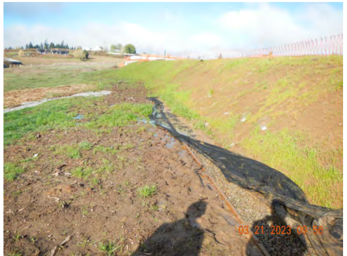
Photo #:08 (DSCN3168) Description: Facing west, photo of the discharge area from the southern stormwater pond (Tract G). Stormwater discharges from the pond to a dispersion trench, to the neighboring property/vegetative area.
