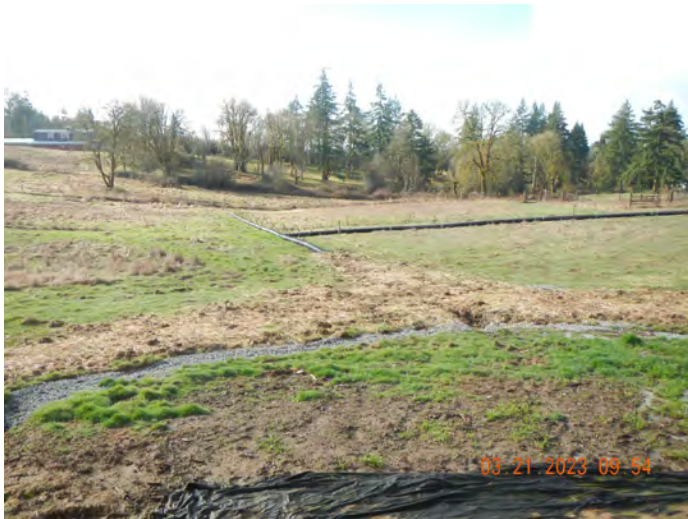
Photo #:07 (DSCN3167) Description: Facing south, photo of the discharge area from the southern stormwater pond (Tract G). Stormwater discharges from the pond to a dispersion trench to the neighboring property/vegetative area.
