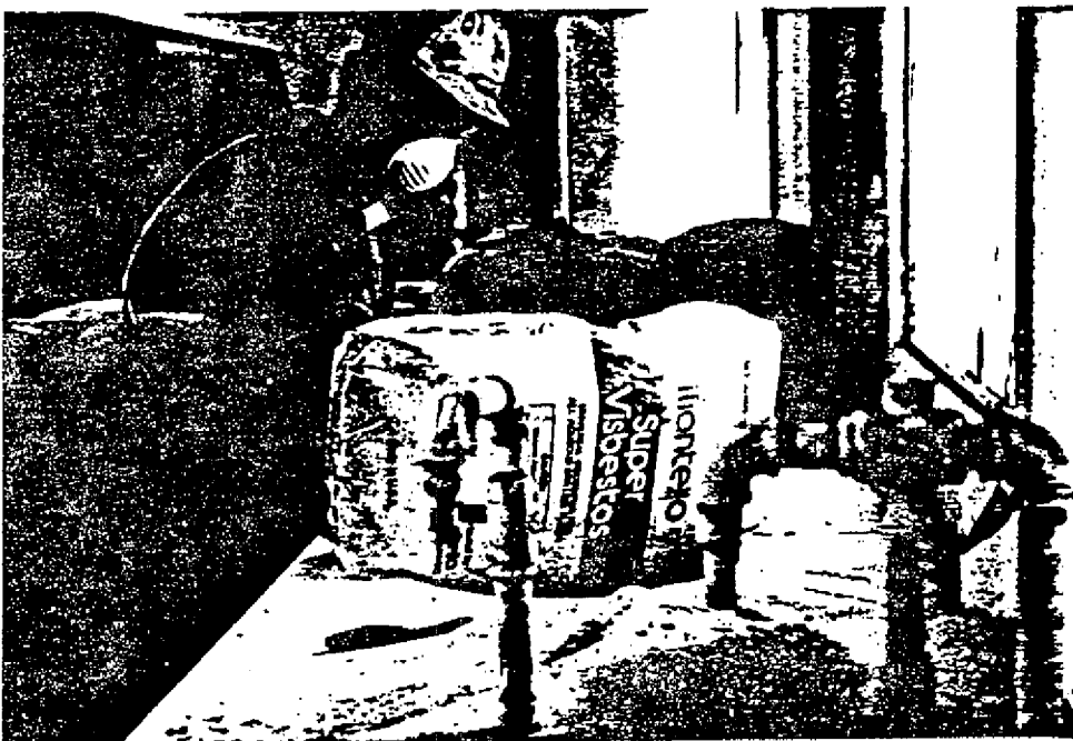
Photograph #4 - Operator continuing to add "Supervisbestos"
