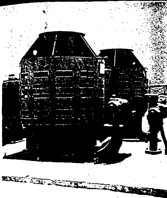
Caught in a snowstorm are the two Elliott 500-hp, 440-rpm, vertical weather-protected motors which drive the circulating water pumps for unit No. 1. The location is at the river.
