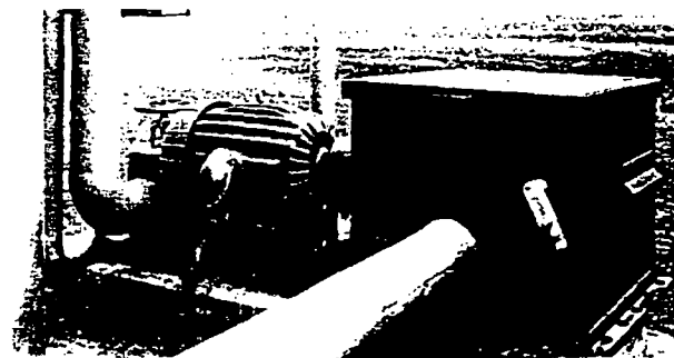
Above—Closeup of Elliott C-W motor driving traveling water screens. Below—20-hp, 3600-rpm motor driving clearwell water pump outside water treatment building.
