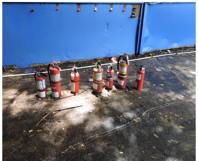
Picture 20 - DCN RECYCLING, CORP. - As observed at the Machine Shop Area , there were approximately seven (7) discarded extinguishers placed on the concrete floors without any containment measures or labels.
