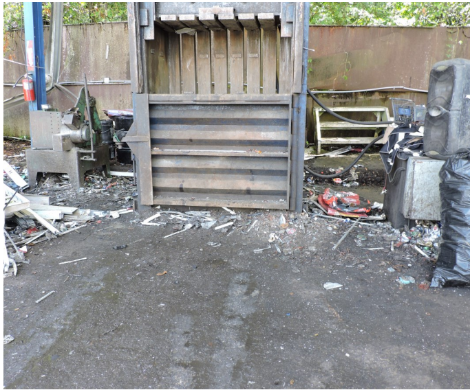
Picture 17- DCN RECYCLING, CORP. - As observed by the EPA Inspector at the Compacting Aluminum Accumulation Area, there were leaks incidents on the concrete floor that appears to contain used oil from crushing machines and heavily impacting soils in the backyard with used oil.
