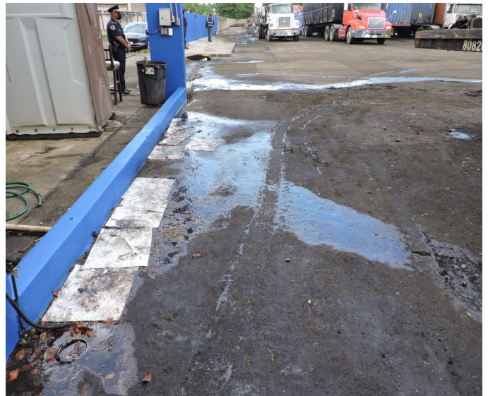
Picture 30 - DCN RECYCLING, CORP. - As observed during the EPA Inspection, there were run-offs from the Facility were accumulated at the Fuel-Oil Station during rain events and were discharged directly toward a nonfunctional sump and then into the sidewalk curb nearby water creek located northwest of the property edge.
