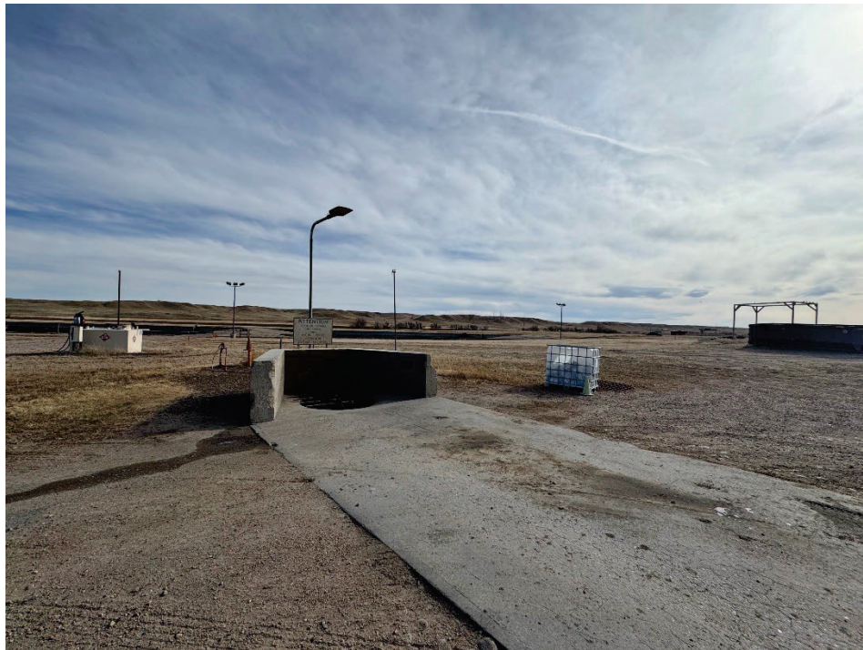
Figure 7 – Dry Creek POTW Septic Disposal Station
