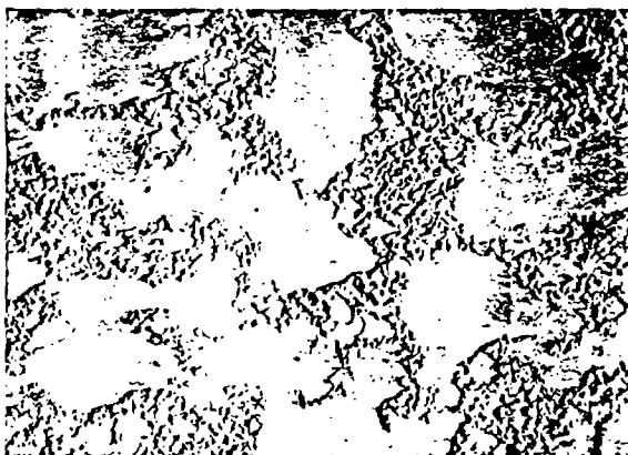
MODERN CALIFORNIAN Stippled— medium heavy dash—flat- tened vigor- ously with trowel
