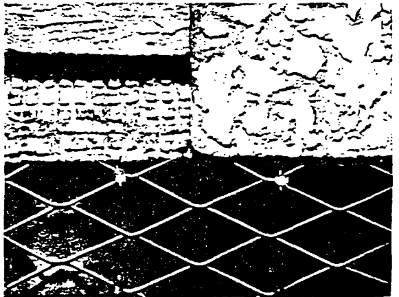
EXPANDED STUCCOMESH —Diagonal strands provide distribution of steel to overcome initial shrinkage, temperature changes, wind stress-protection against unusual snocks.
