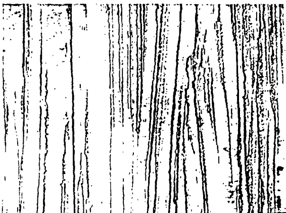
VERTICAL GRAIN Vertical brush- ing—flattened with vertical trowel strokes
