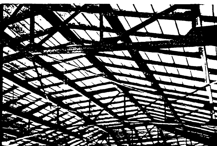
Underside of Sheetrock Pyrofill roof, illustrating the high light reflection quality of this construction.
