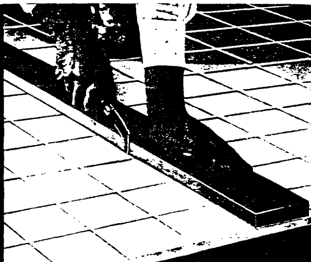
Odd-sized pieces are easily cut from standard sized boards.
