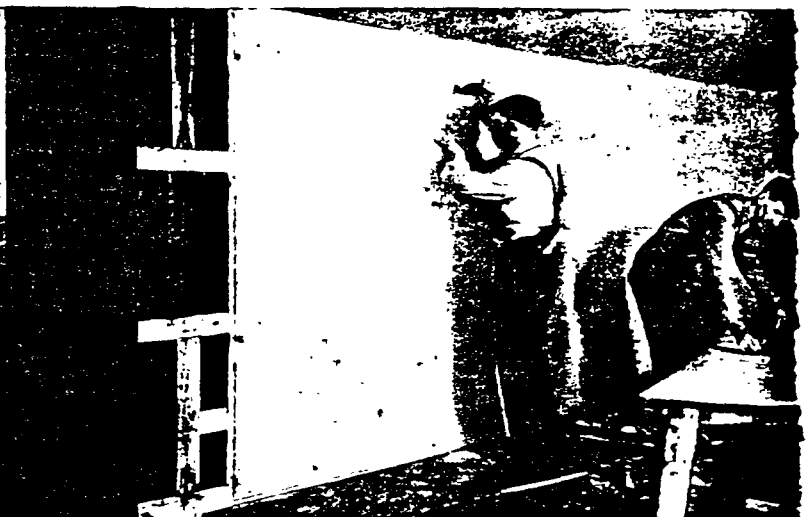
Large sheets permit speedy erection.
