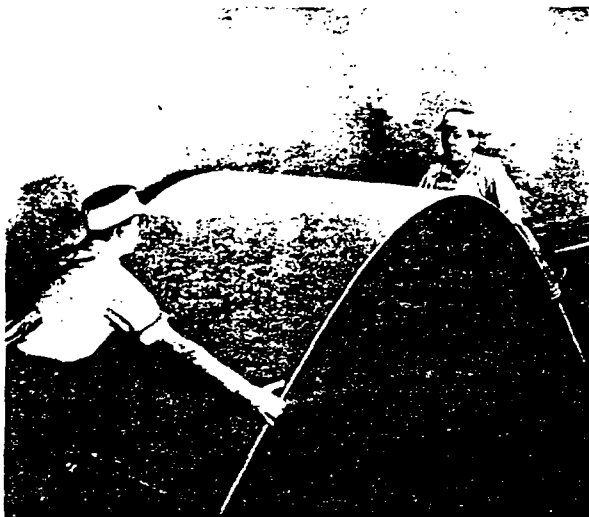
Flexibility of Sheetrock adapts it for use on curved surfaces.
