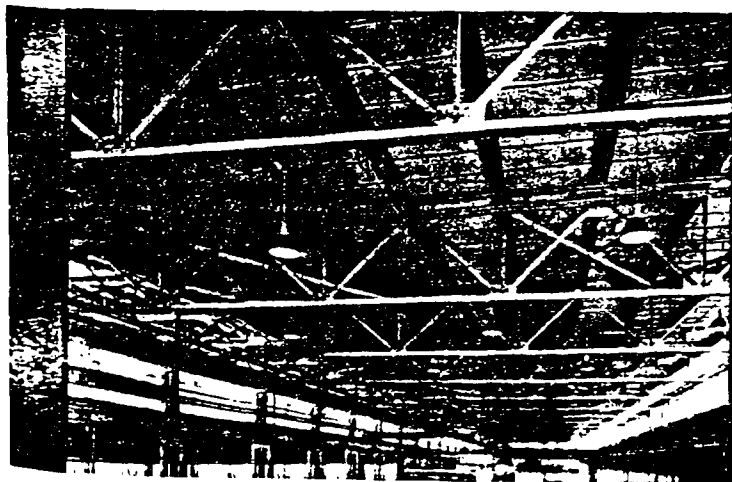
Pyrofill construction is adaptable to any type of steel framing or truss construction.
