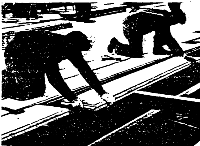
Tongue and groove edges permit USG Gypsum Plank to cantilever. Therefore, ends do not have to meet over supports.
