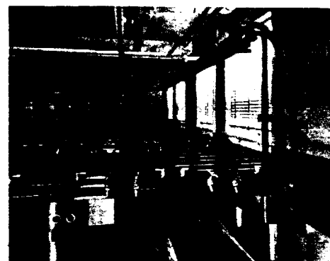
The Hancock Foundation Building, University of Southern California, uses lead pipe and valves for salt water lines
