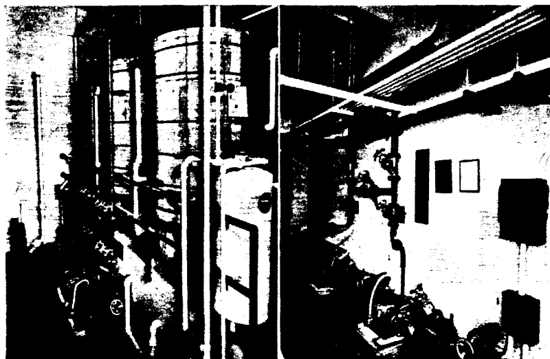
At far left, pumps, hard lead pipe and angle valves. Left, distributing pumps, hard lead valves and pipe in the filter room. Note brackets and horizontal supports
