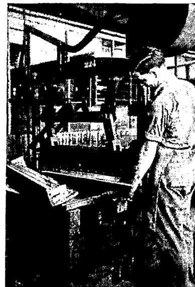
Fig. 4. Left hand on air valve. Right hand moves stock through pulley arrangement.
