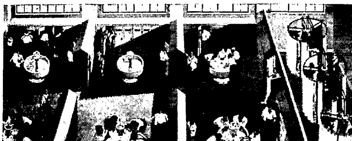
Installation of Bradley Washfountains and 5-Unit Showers
