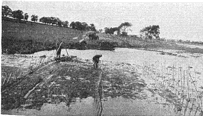
Left—Just before a blast was set off on the Bristol-Fall River Highway job. Note the three rows of pipes, marking the location of charges loaded in the holes
