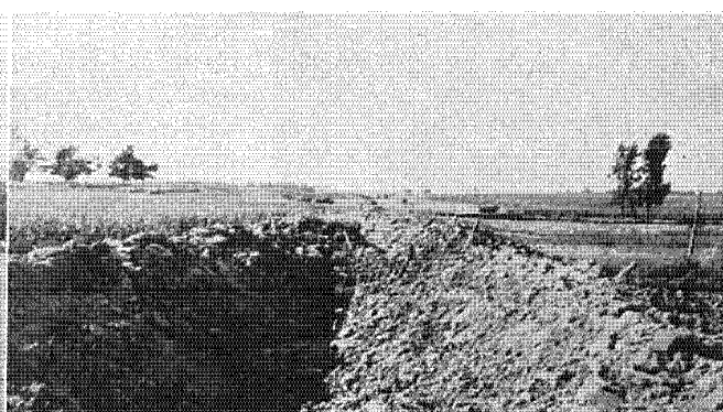
Right—After the blast. This shot displaced the unstable material so that the central area of a nine-foot embankment dropped down to the clay bottom
