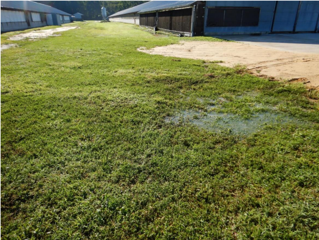
Photograph 11. View of standing water located 30-40 ft northwest of Poultry Barn 1.
