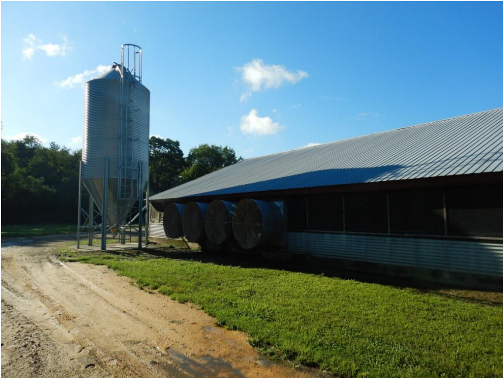
Photograph 3. View, looking southeast, of the exhaust fans and feed storage bin located on the northeast corner of Poultry Barn 1.
