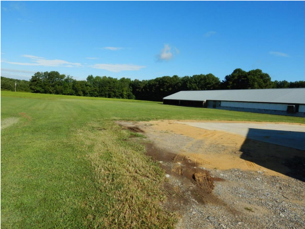
Photograph 19. View of the concrete pad on the west end of Poultry Barn 1 with Poultry Barn 2 visible in the background.
