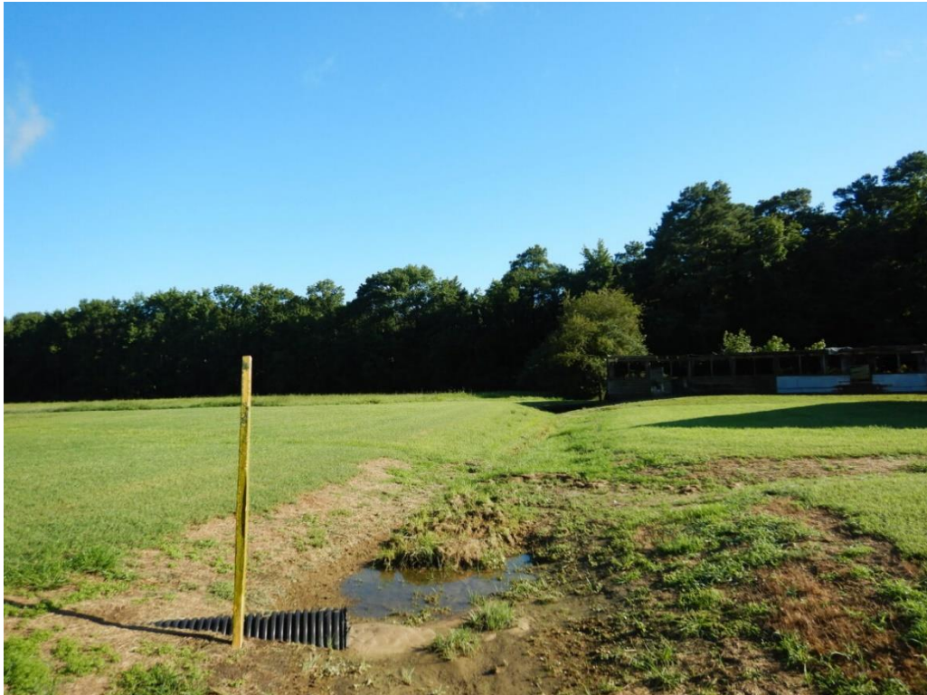
Photograph 5. View of a culvert that outlets into the swale shown in Photograph 4. The swale directs flow towards the northern boundary of the facility.
