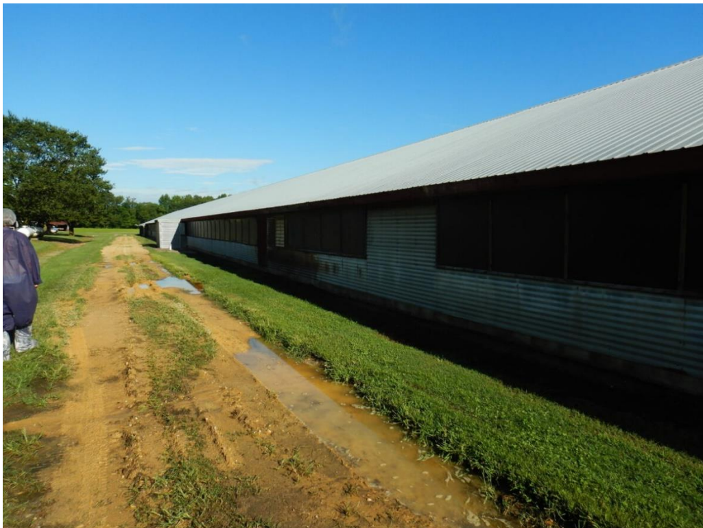
Photograph 16. View along the south side of Poultry Barn 1.
