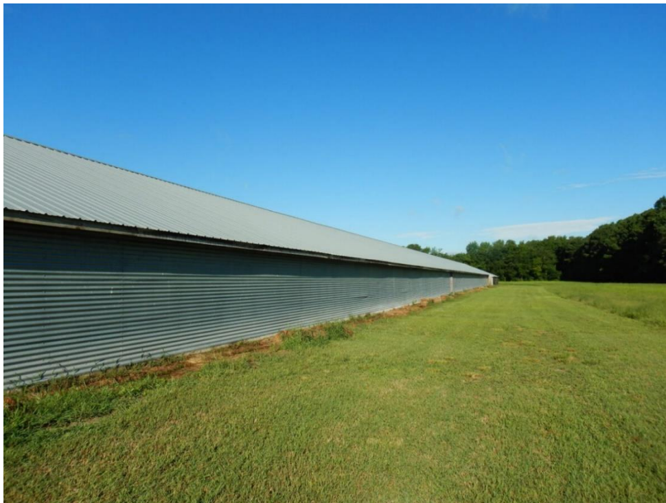
Photograph 8. View facing west along the north wall of Poultry Barn 2.
