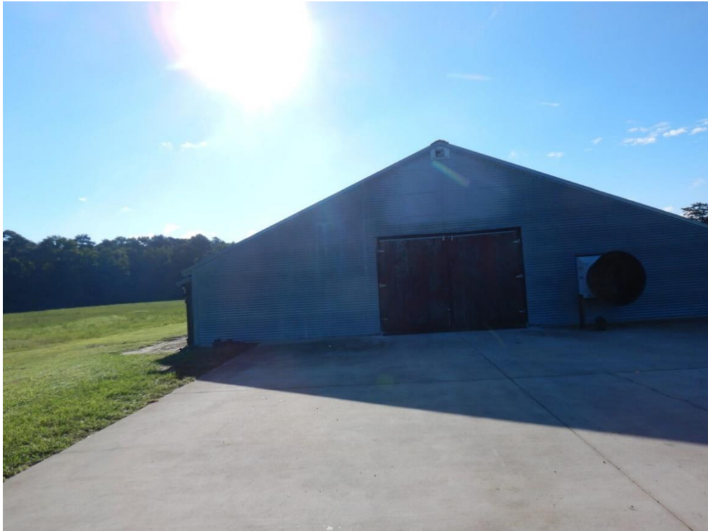
Photograph 9. View of the west side of Poultry Barn 2 and the barn's concrete pad.
