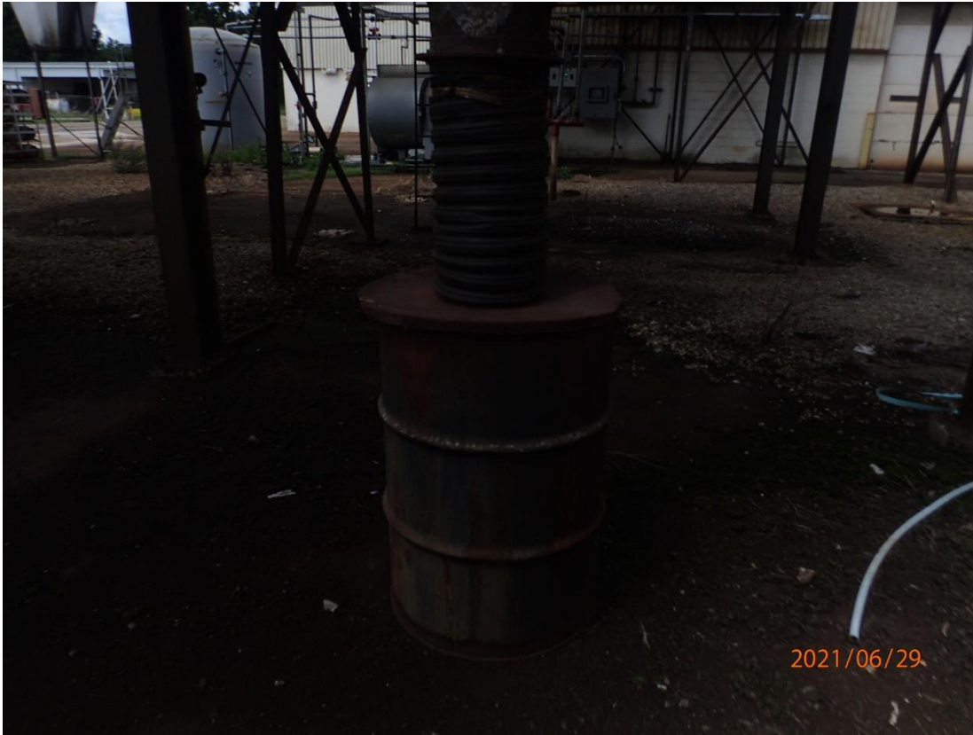
Photo 13: Second 55-gallon container attached to a baghouse. The container was not labeled.
