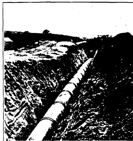
COURTESY U. S. PIPE & FOUNDRY CO. A section of the 36 in. cast iron pipe line that has 11,000 poured lead joints
