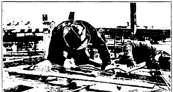
Installing sheet lead, showing "burning" or welding in process
