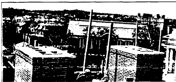
Two lead covered chimneys with rain-water vents
