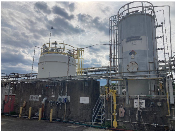
Photograph 9: Hazardous waste tank CAA.
