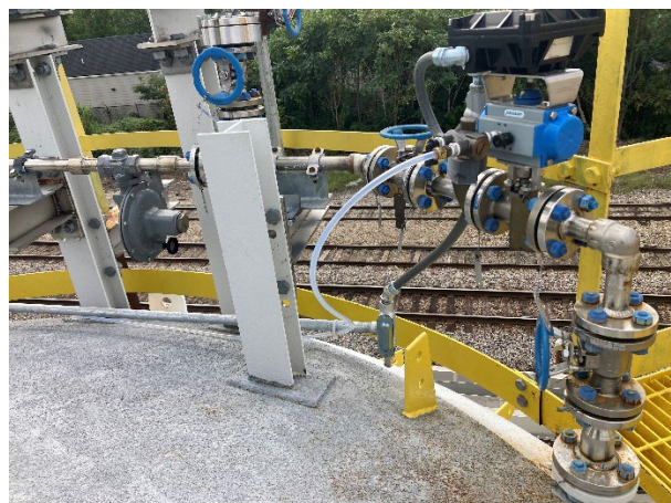
Photograph 16: Hazardous waste tank CAA.
