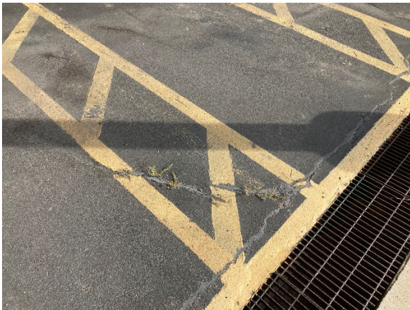
Photograph 8: Floor of Hazardous waste container CAA.
