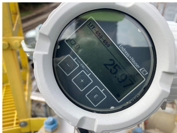
Photograph 15: Hazardous waste tank CAA.
