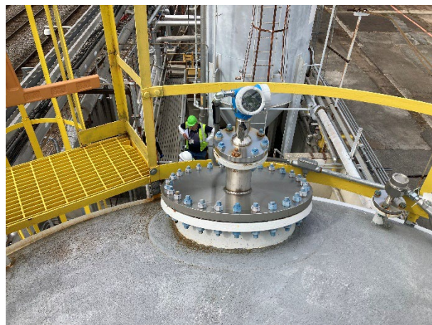
Photograph 14: Hazardous waste tank CAA.
