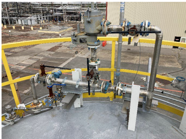
Photograph 13: Hazardous waste tank CAA.
