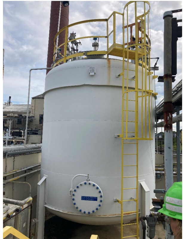
Photograph 10: Former Hazardous waste permitted tank.
