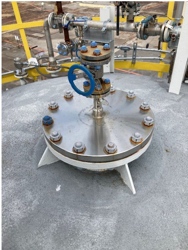
Photograph 12: Hazardous waste tank CAA.
