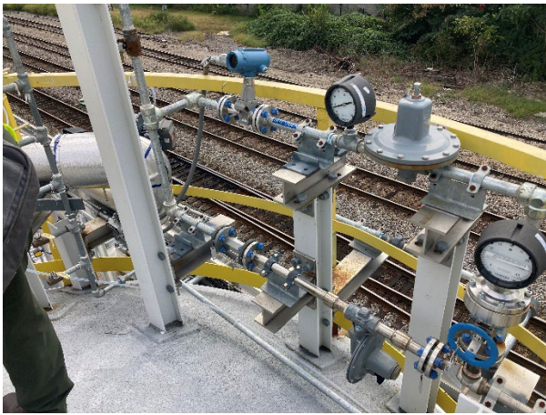
Photograph 17: Hazardous waste tank CAA.
