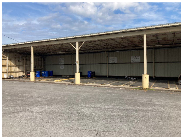
Photograph 1: Permitted Container Storage Area and CAA for containers.
