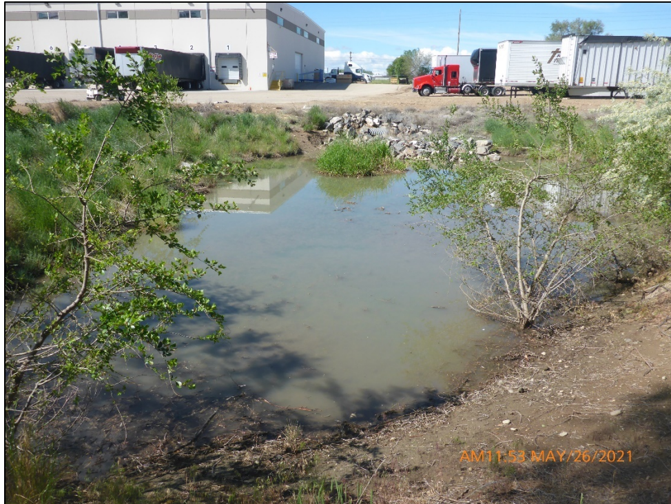
Photograph 15. Additional view, facing southwest, of the stormwater retention basin shown in Photograph 14. Note the basin has standing water from a storm even that occurred the night before.
