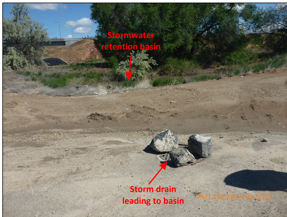
Photograph 14. View of the stormwater retention basin and associated storm drain in the northeastern portion of the northern parcel.
