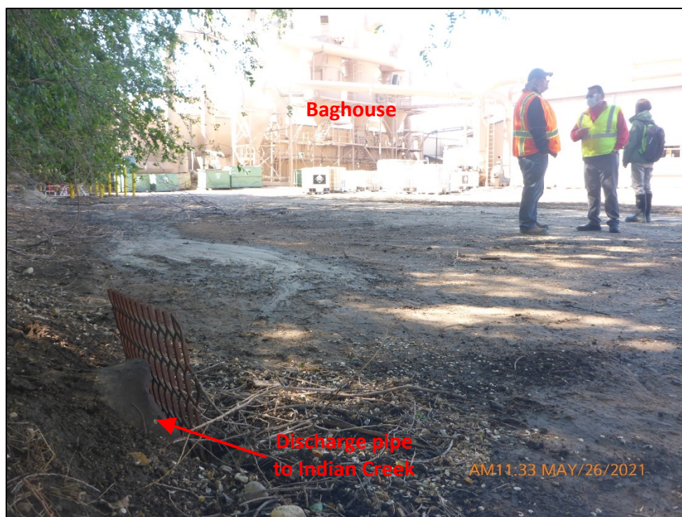
Photograph 17. View of the baghouse located upgradient of the unnamed open pipe stormwater discharge point (shown in Photographs 6 and 7) south of Outfall SW1.
