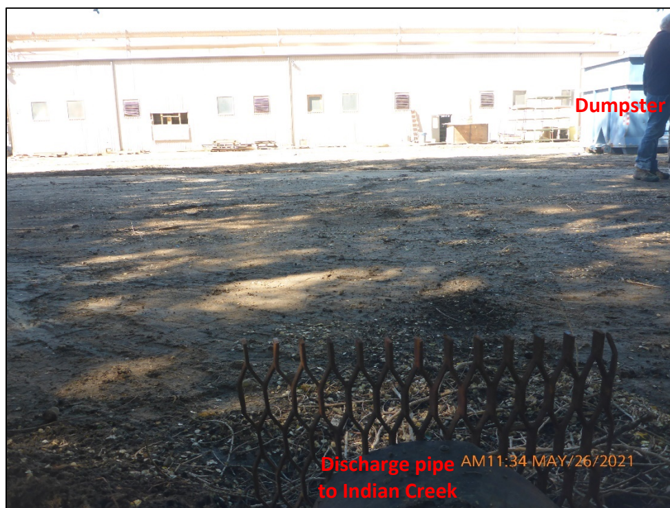
Photograph 18. View of the waste dumpster located upgradient of the unnamed open pipe stormwater discharge point (shown in Photographs 6 and 7) south of Outfall SW1.
