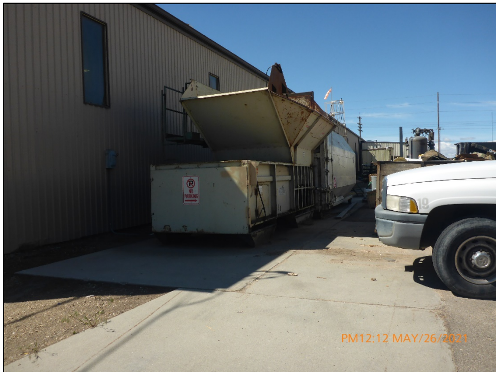
Photograph 26. View of the trash compactor upgradient of the storm drain shown in Photograph 5. This trash compactor was not identified on the SWPPP site map provided by the Permittee.
