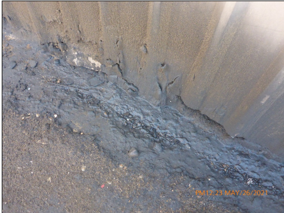
Photograph 25. Close-up view of the dark residual staining shown in Photograph 24.
