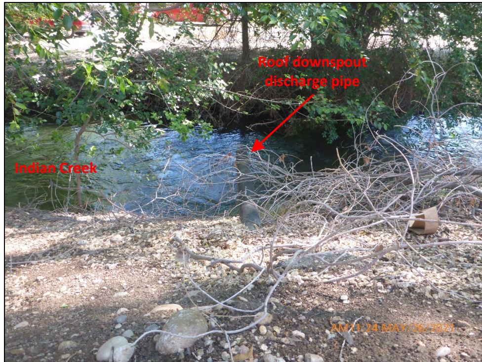
Photograph 11. View of the discharge pipe to Indian Creek from the roof downspout shown in Photograph 10.
