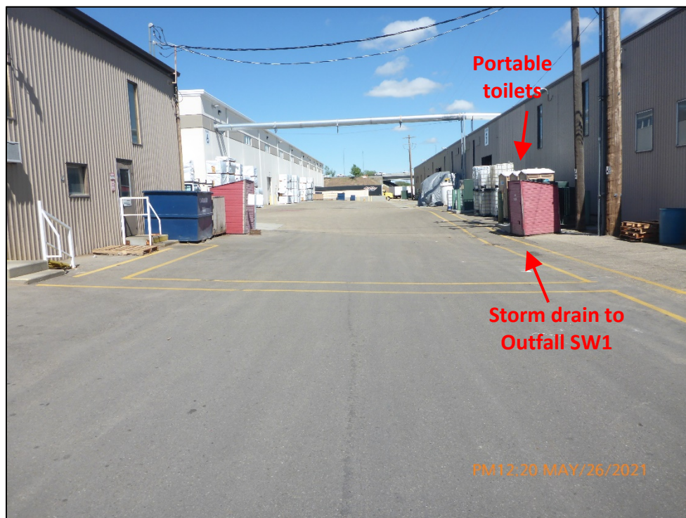
Photograph 4. View of a storm drain located in the central portion of the northern parcel. This storm drain flows through a sand/oil separator and to Outfall SW1 shown in Photographs 2 and 3. Note the portable toilets adjacent to the storm drain which were not on the site map.
