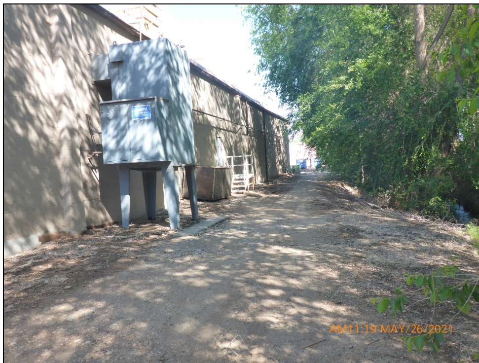
Photograph 9. View, facing northwest, along the Facility's southeast perimeter with Indian Creek. Multiple roof downspouts from the warehouse building are piped underground to Indian Creek. Other discrete overland conveyance discharge points were also observed in this area.
