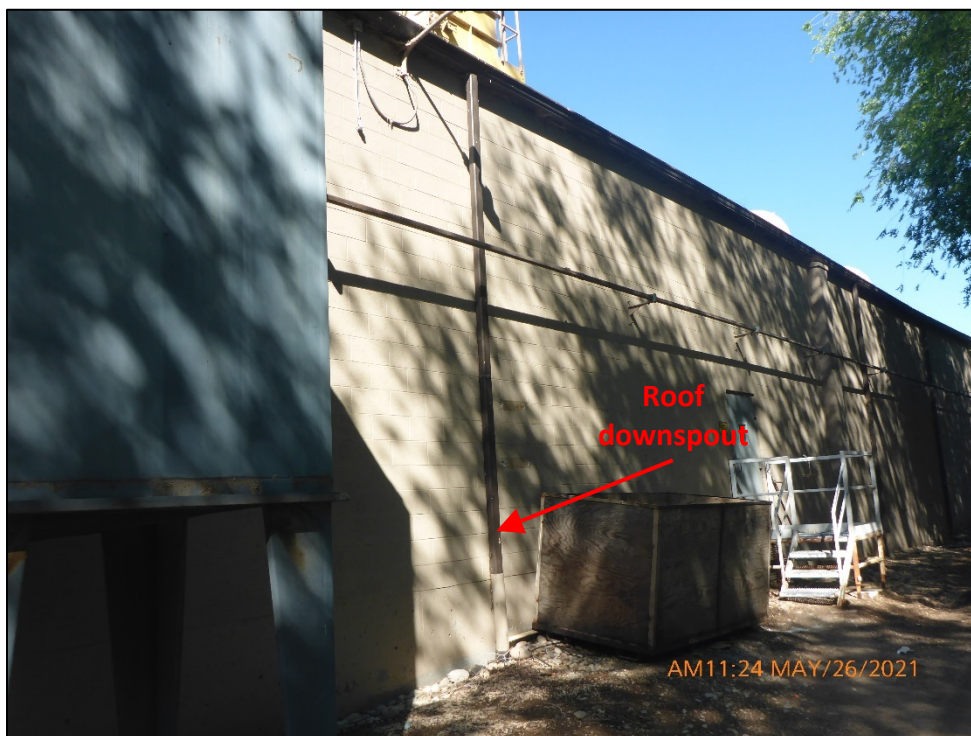
Photograph 10. View of a roof downspout on the warehouse building shown in Photograph 9. This downspout is piped underground to Indian Creek (as depicted in Photograph 11).
