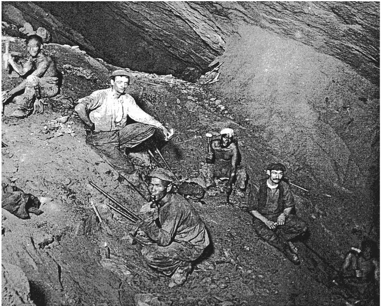
Taking out the foot wall the old way, and probably contacting miners' phthisis at the same time.
