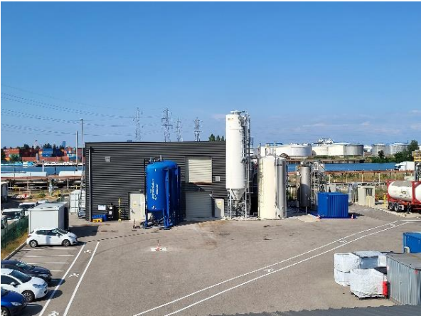
Current waste water plant
