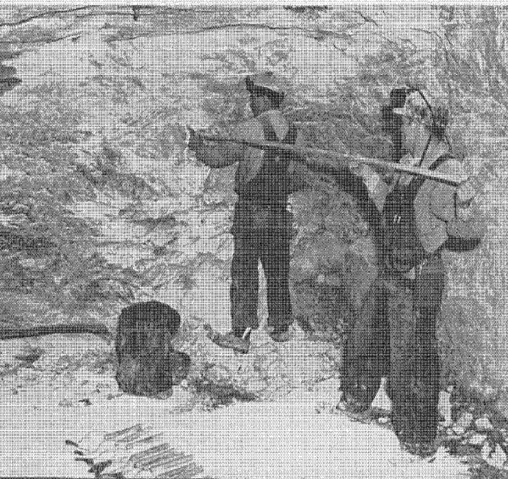
◀ After ore is removed, the mine face is undercut, drilled again and loaded with Du Pont dynamite.
