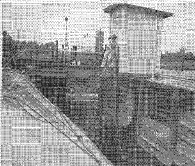
Plant's liquid waste is treated to avoid polluting stream. Sample being taken here is check on treatment's efficiency.
