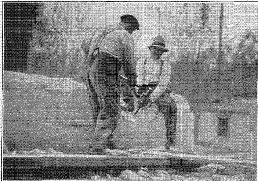
This slow, tedious detail of battering down a concrete wall by hand with high-priced labor could have been avoided by the use of a few small charges of dynamite. Any danger to adjoining buildings can be avoided by careful loading and the use of blasting mats or timbers.
