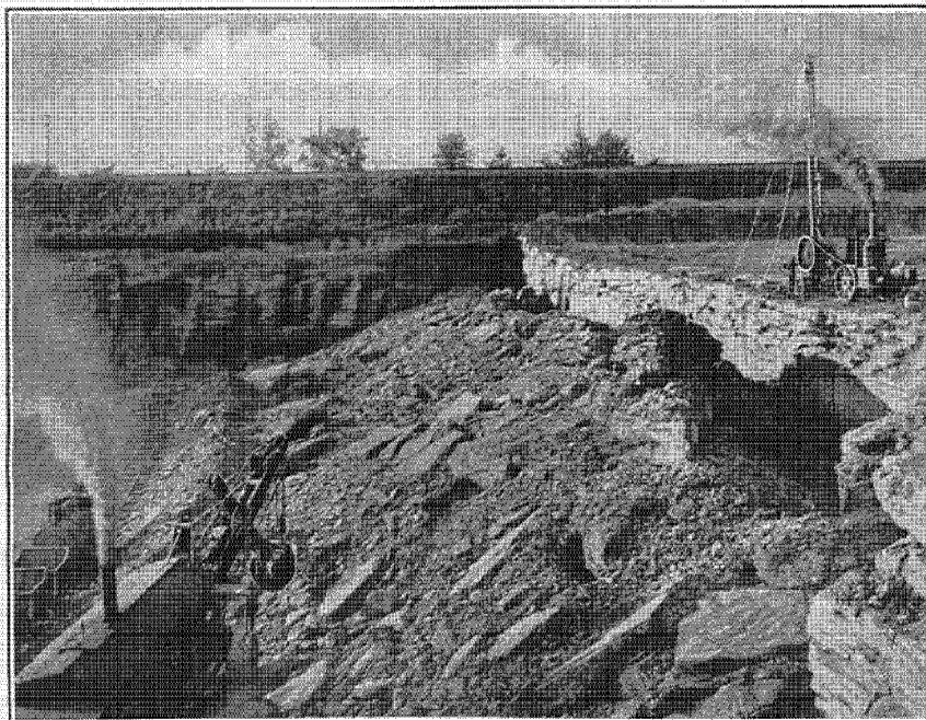
Fig. 5—A Buffer Shot; Broken Stone is Left in Place to Prevent Fragments Flying from the Next Blast
