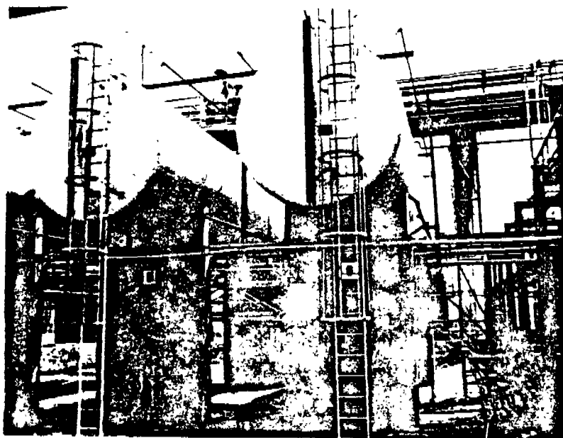
Figure 3.20 Cylindrical, side-by-side, above ground VC storage tanks are shown. RD/SRV vents may be seen on pipe rack above tanks.
