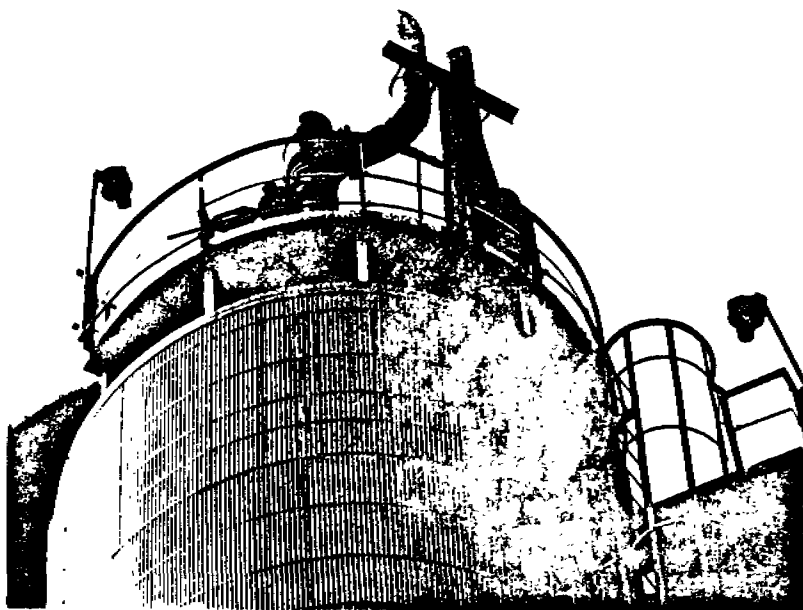
Figure 3.31 An EDC finishing column with the RD/SRV and its vent mounted on the top. (In some installations the finishing column performs the function of the light ends distillation column while in others it encompasses the functions of both the light and heavy ends columns.)
