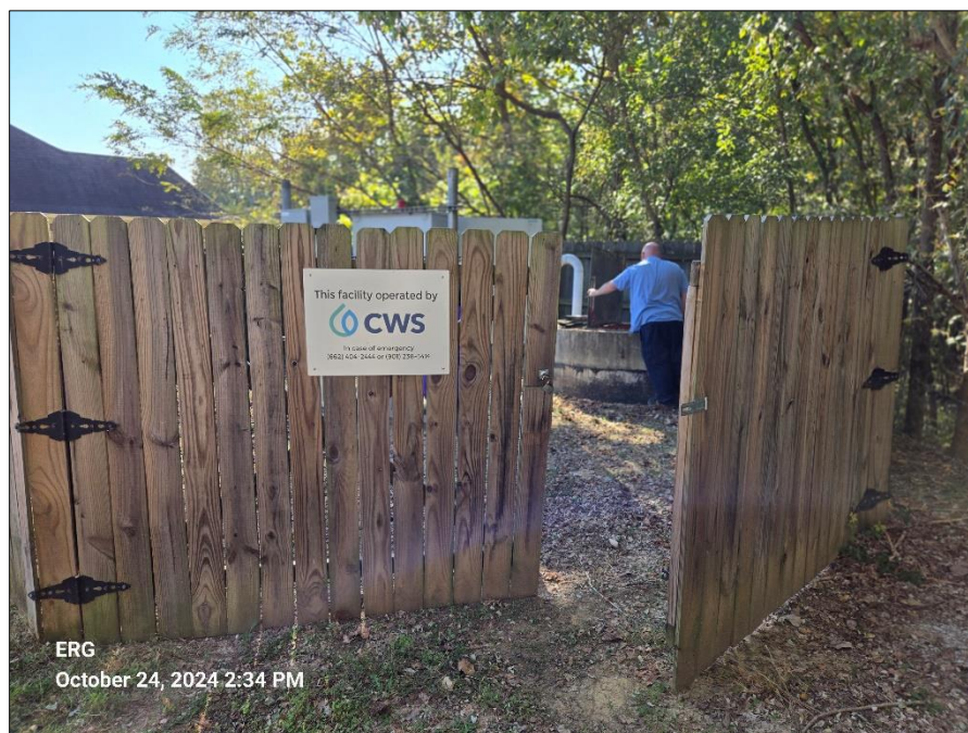
Photograph 6. Morningside lift station perimeter fencing.
