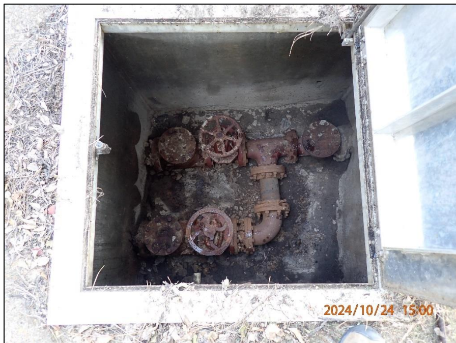
Photograph 16. Railroad lift station valve pit.
