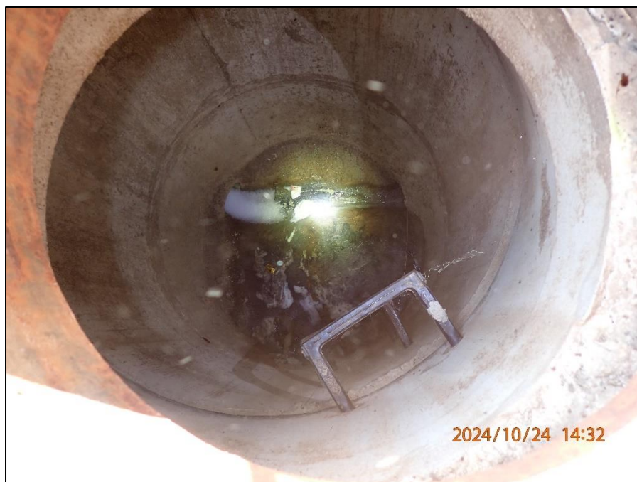
Photograph 5. Interior of the Morningside manhole.
