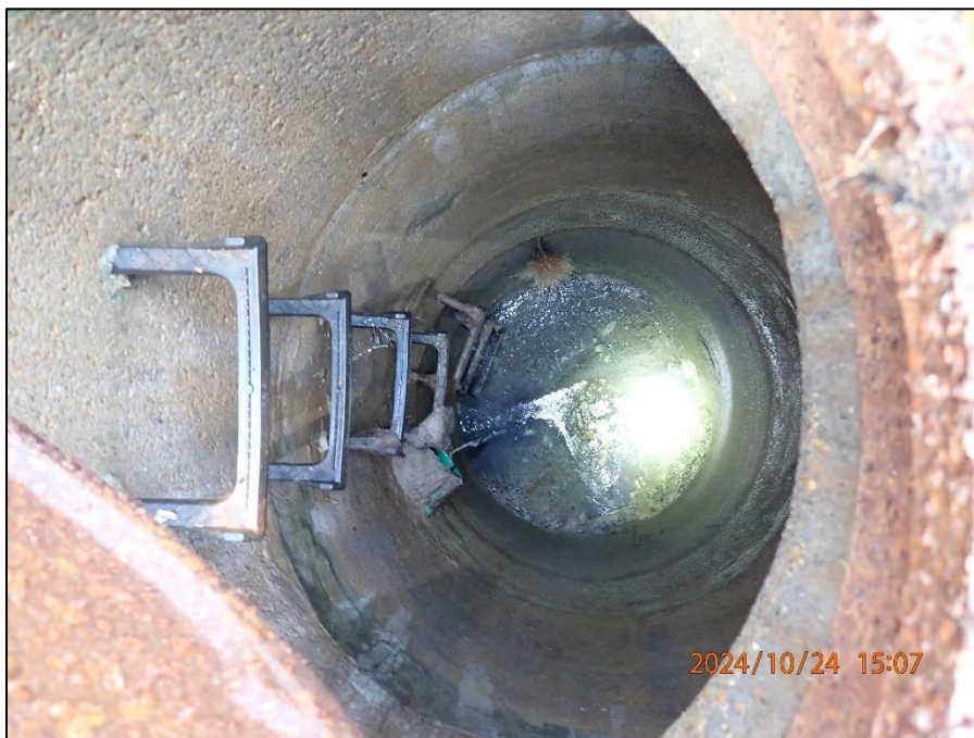
Photograph 18. Interior of the Railroad manhole.
