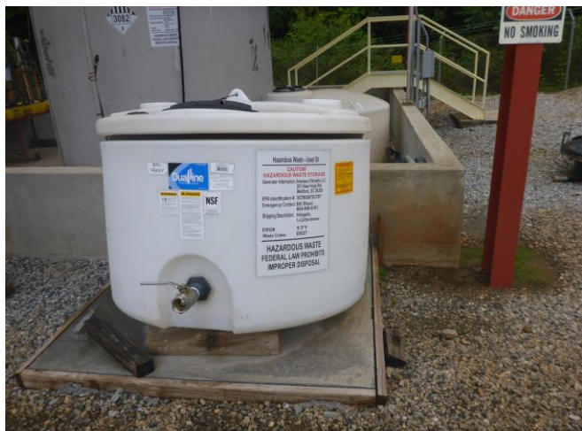
Photo 7 – Hazardous Waste Tote: 300-gallon tote used to accumulate oily liquid waste (D001, D009, D027).
