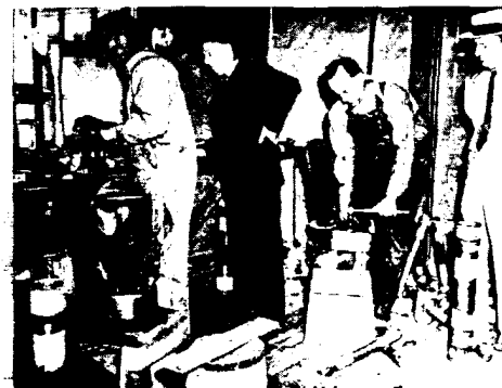
Bottom, journeyman prepares lead pipe for wiping while plumbing inspector Kissling and O. B. Monier look on
