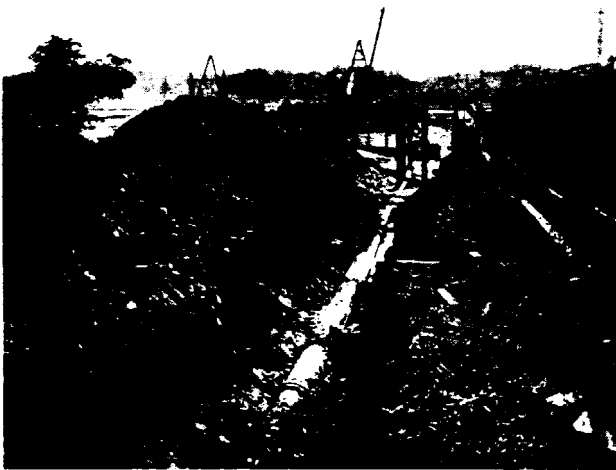
A section of the submarine line suspended by rope and chain falls before lowering into the water in sections of about 100 ft. long and already calked together
