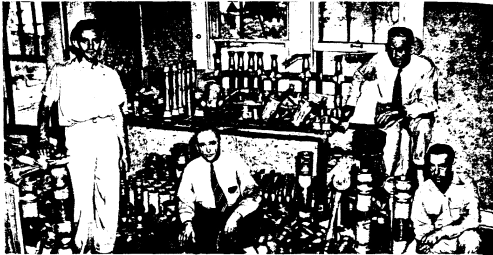
Left to right, kneeling, A. J. Monier, president, and O. B. Monier, vice-president, of A. J. Monier, Inc., plumbing contractor for Alazan Courts Housing Project: standing, Kurt A. J. Monier, secretary-treasurer, and Oran J. Vick, plumbing inspector on the project
