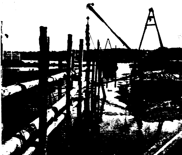
A section of the submarine line suspended by rope and chain falls before lowering into the water in sections of about 100 ft. long and already calked together
