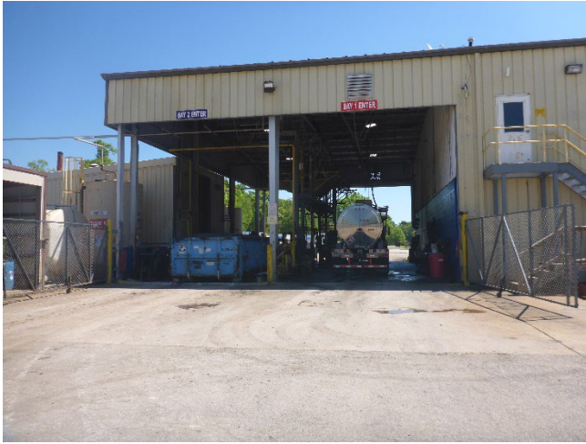
Photo 4: Two truck wash bays.
