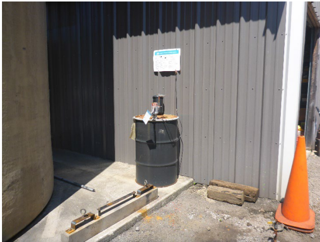
Photo 1: SAA for managing the contents from punctured aerosol cans. The drum was not labeled with the words hazardous waste or marked with an indication of the hazards of its contents. The bung on the drum was equipped with a can puncture device, which was open.
