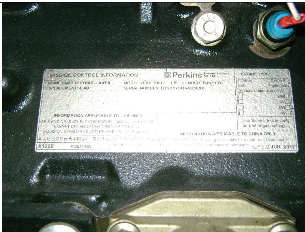
Plate on emergency generator engine.
